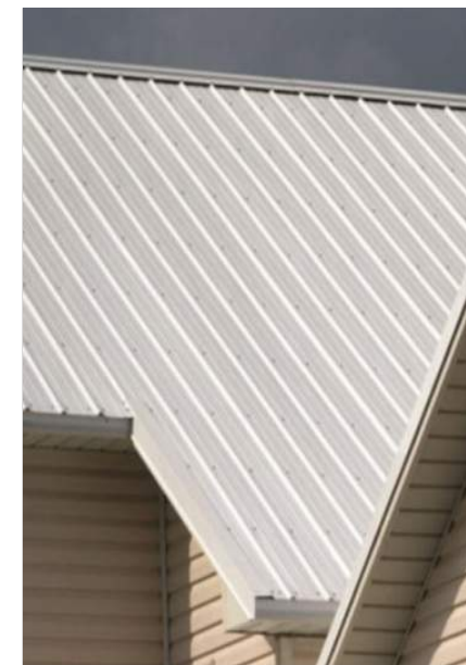
PAC Clad standing seam metal roof in Stone White on shed roof and east elevation. Matching color on fascia. Product rated as highly reflective/Energy Star.
