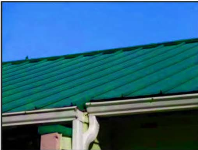
Typical roof drain gutters.
