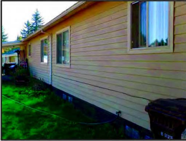
Typical apartment unit exterior wall finishes.
