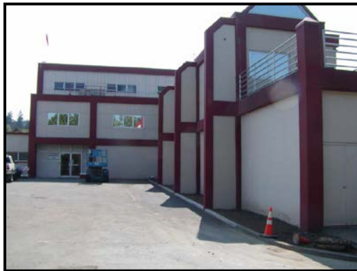
Clackamas River Water Seismic Retrofit Project -Left side: Buttress walls added to treatment plant. Right side: Reservoir wrapped with carbon fiber reinforced polymer.
