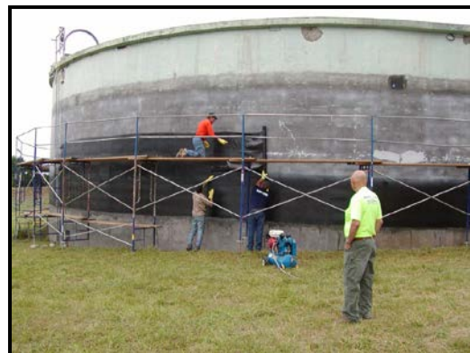
Clackamas River Water Seismic Retrofit Project -Left side: Buttress walls added to treatment plant. Right side: Reservoir wrapped with carbon fiber reinforced polymer.
