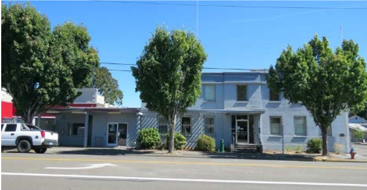
Figure 2. Primary (west) façade of Gladstone City Hall, view northeast (ARG, September 2020).
