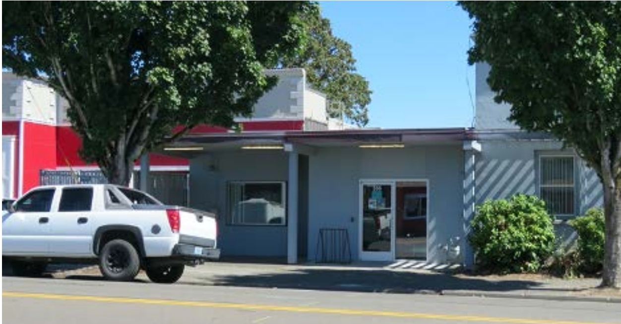
Figure 5. West façade of addition off north façade, view north (ARG, September 2020).
