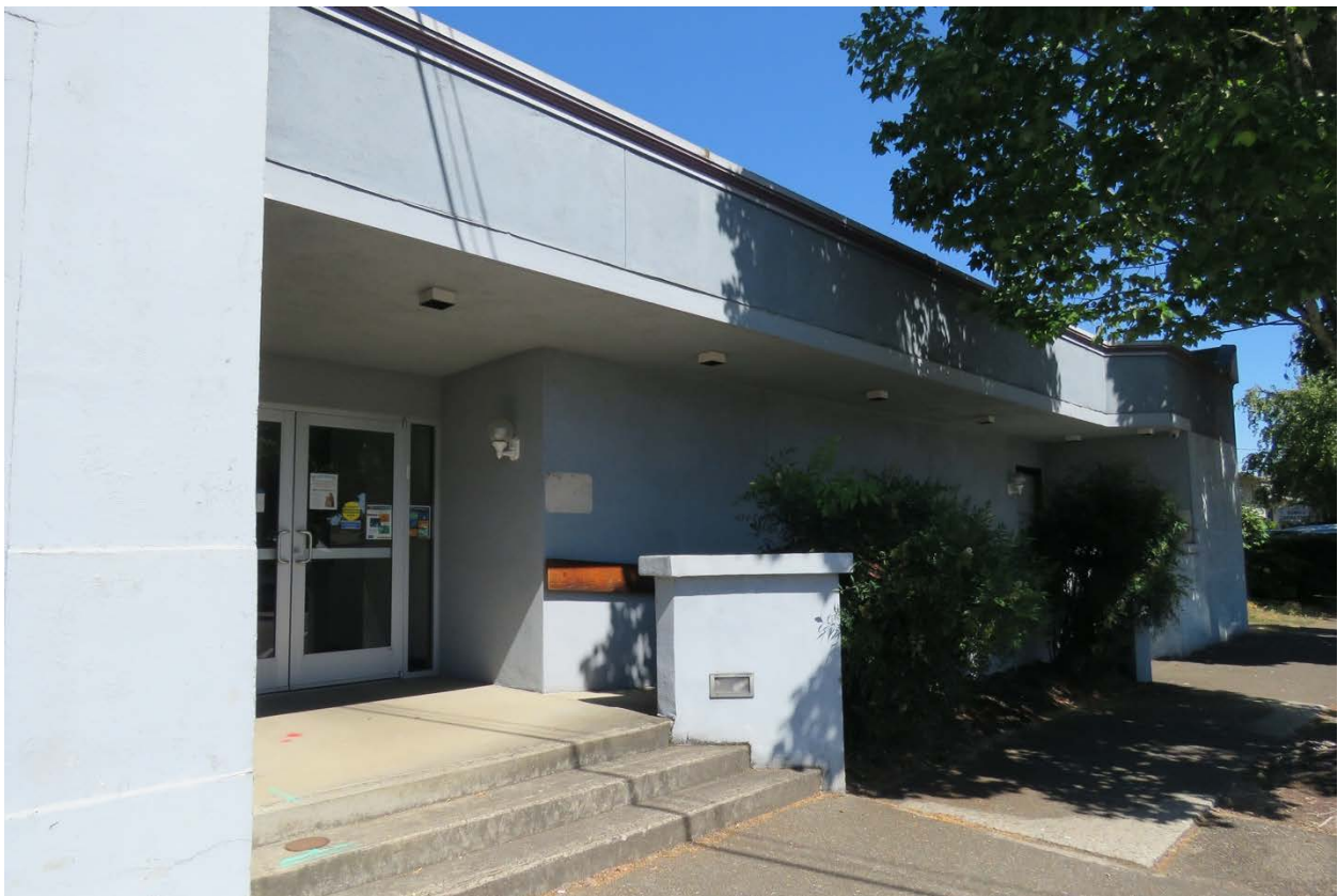
Eastern portion of south façade including two secondary entrances, view north (ARG, September 2020).
