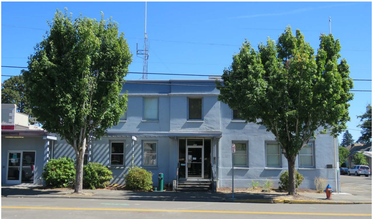
Original portion of the primary (west) façade, view northeast (ARG, September 2020).
