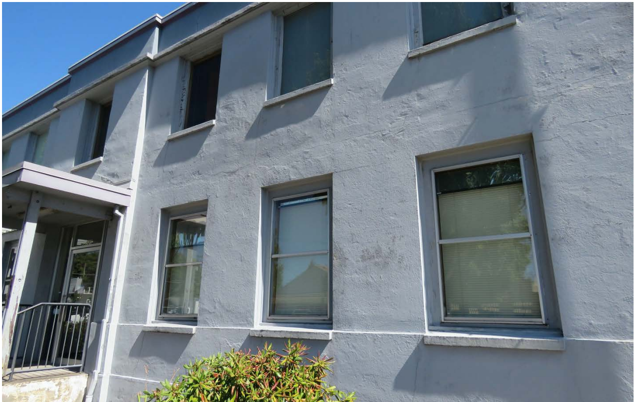
Detail of primary (west) façade showing replacement windows in lower story, view north (ARG, September 2020).
