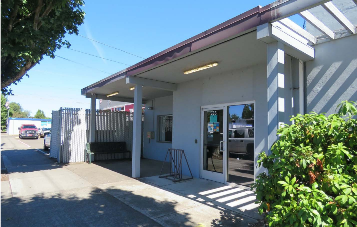
Detail of addition to north façade, view north (ARG, September 2020).
