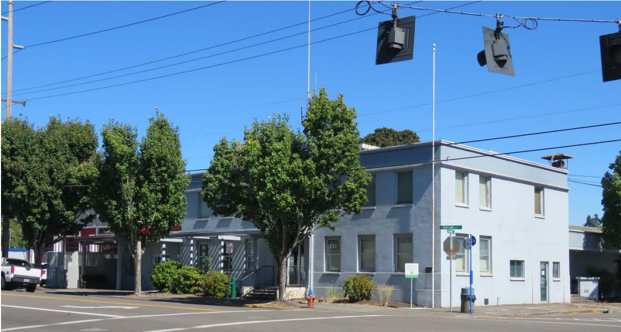
Overview of Gladstone City Hall at 525 Portland Avenue, view north (ARG, September 2020).
