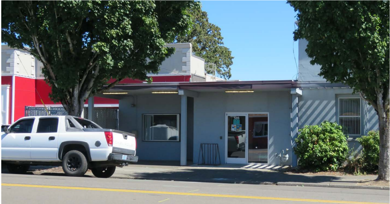
Detail of addition to north façade, view northeast (ARG, September 2020).
