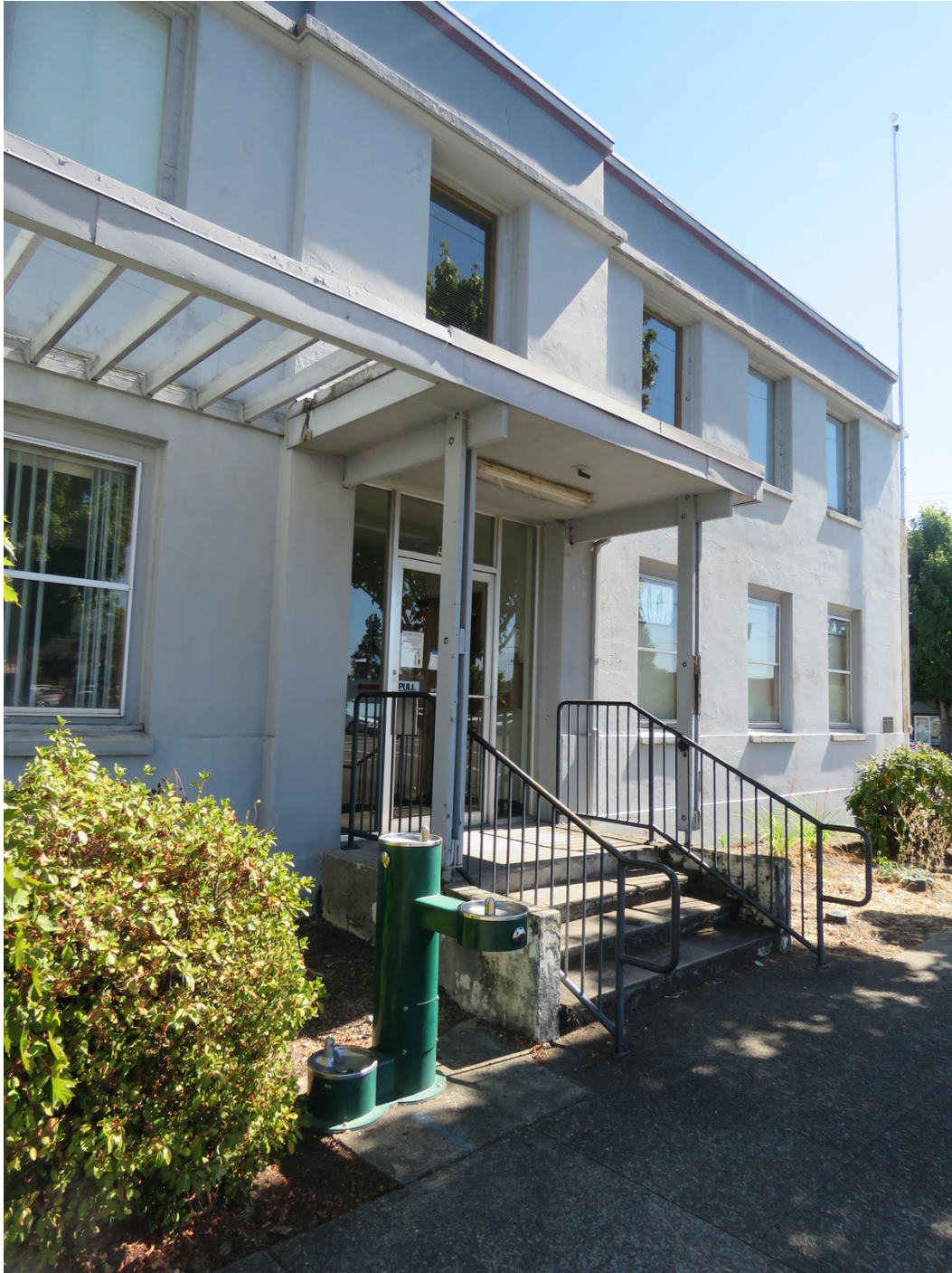
Detail of entrance on primary (west) façade, view east (ARG, September 2020).
