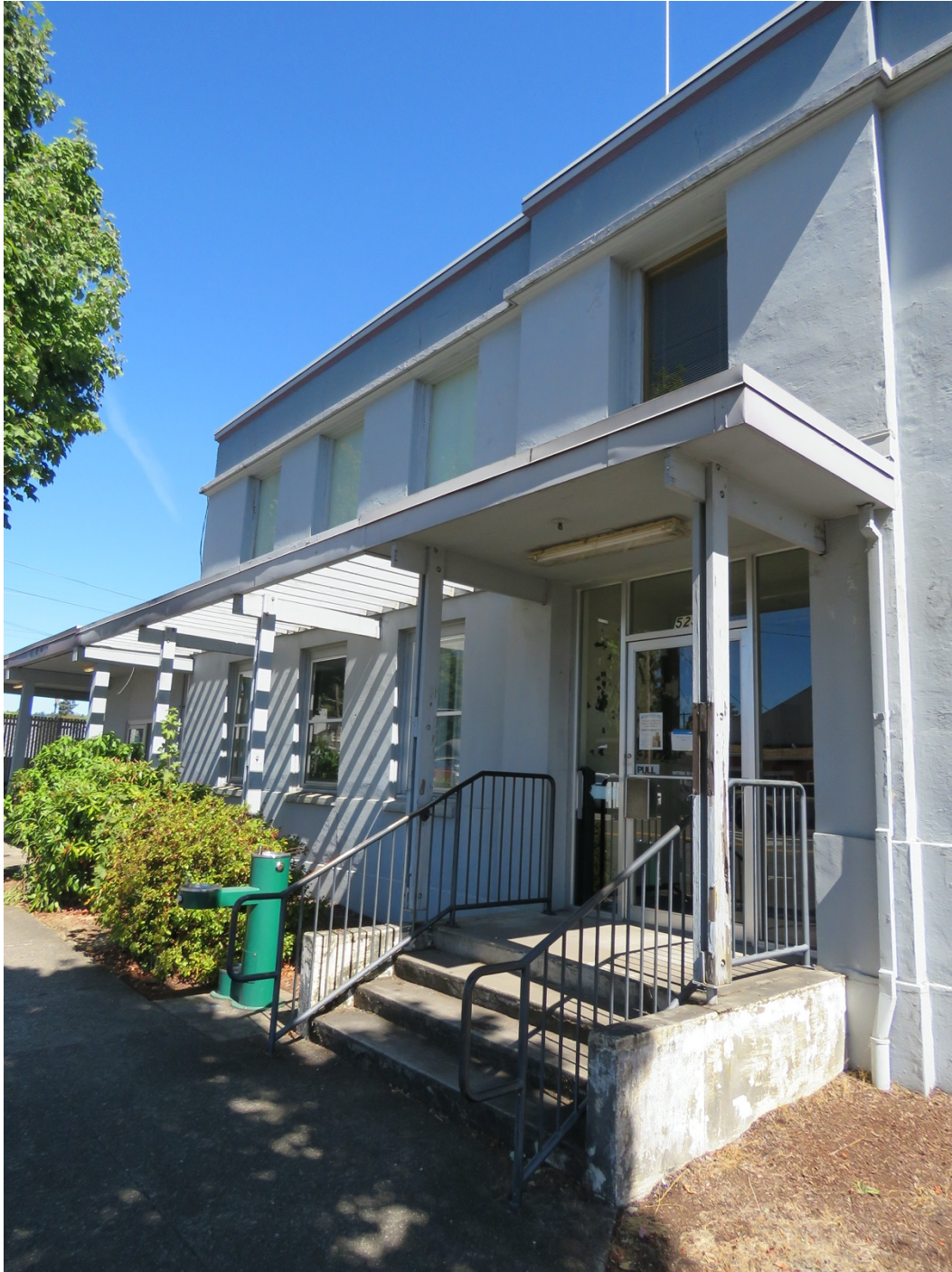
Detail of entrance on primary (west) façade, view north (ARG, September 2020).
