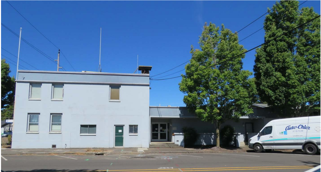
South façade, view northwest (ARG, September 2020).
