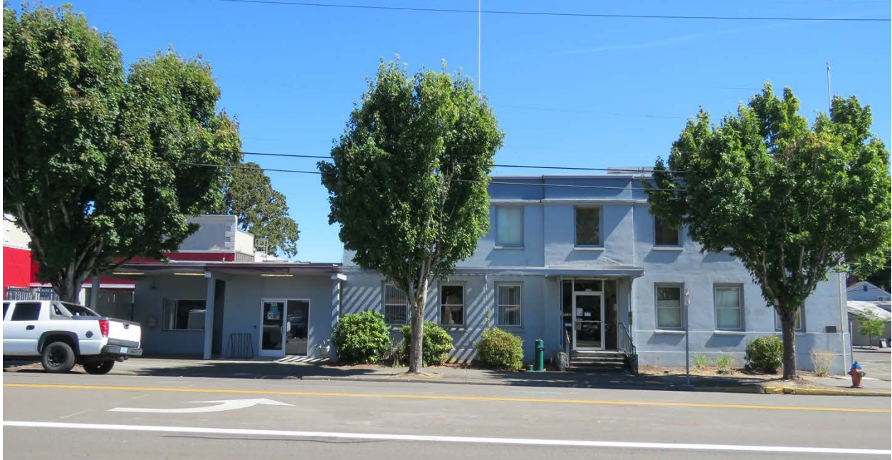
Primary (west) façade, view northeast (ARG, September 2020).
