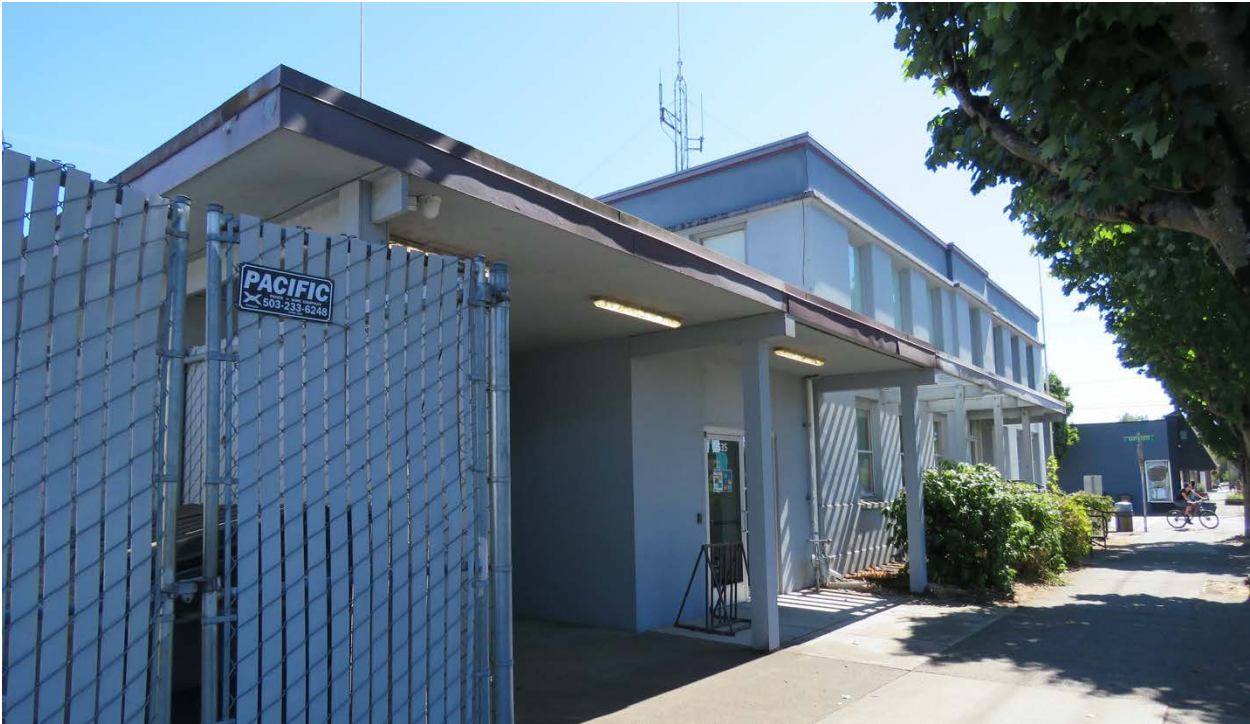
Detail of addition to north façade, view east (ARG, September 2020).
