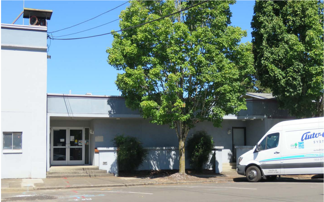
Eastern portion of south façade, view northwest (ARG, September 2020).
