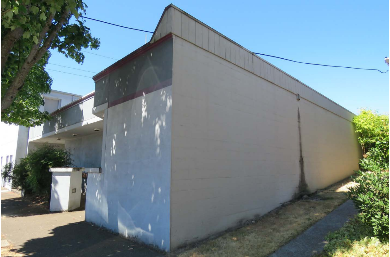
Rear (east) façade, view northwest (ARG, September 2020).
