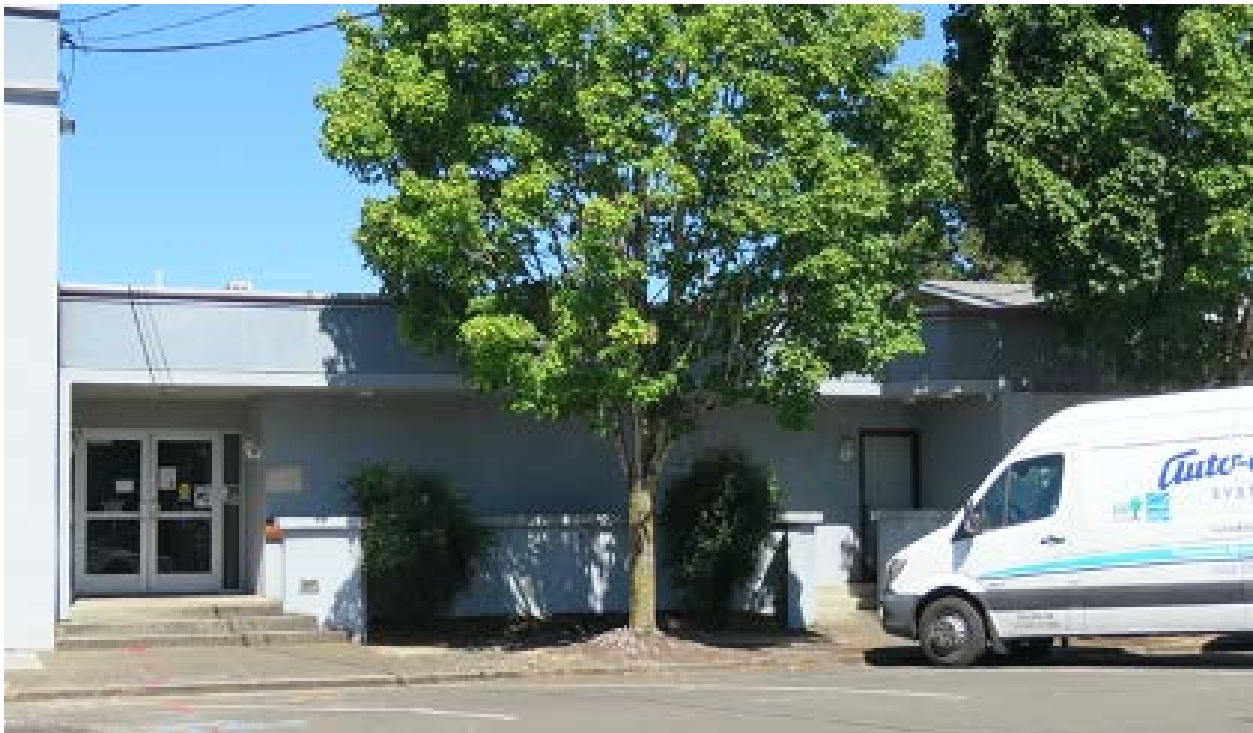
Figure 4. South façade of addition off east façade of Gladstone City Hall, view northwest (ARG, September 2020).
