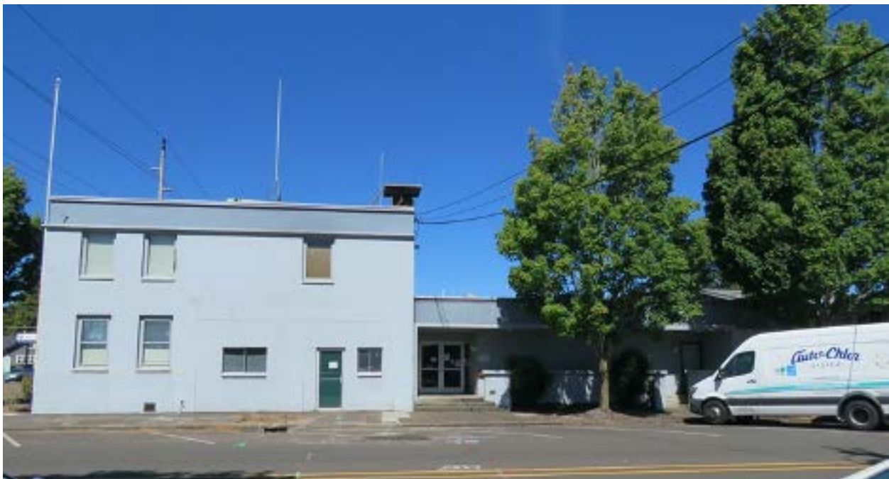
Figure 3. South façade of Gladstone City Hall, view northwest (ARG, September 2020).
