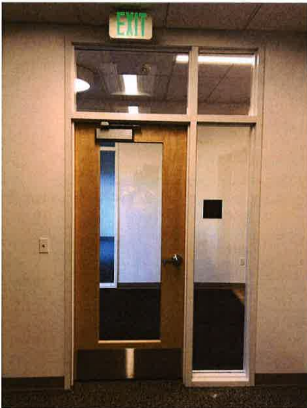
Interior doors, windows & lighting (ground floor)
