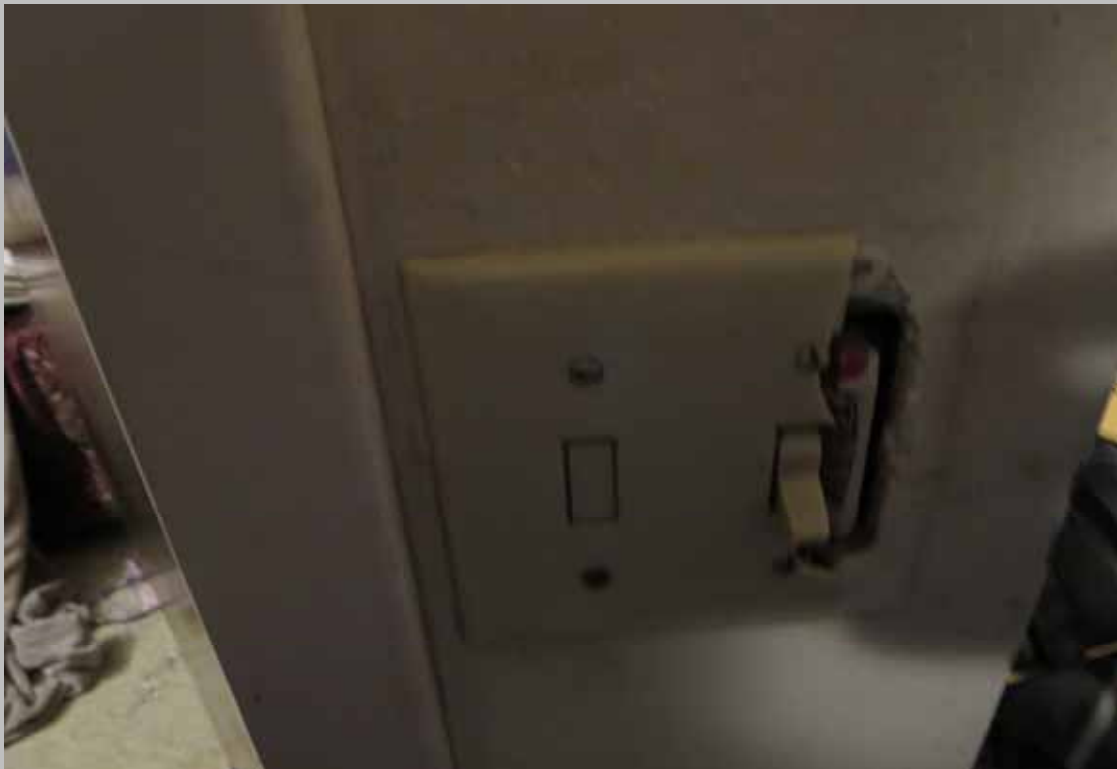
Repair switch cover at unit 903 (Critical Repair)
