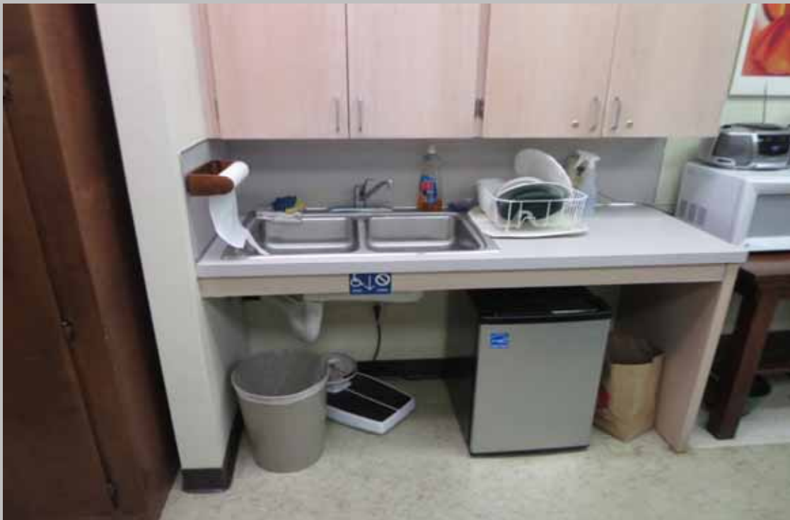
Replace common area cabinets and counters (Non-Critical Repair)
