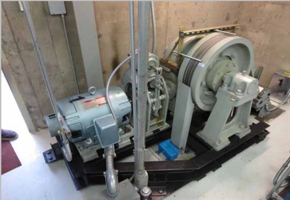
Elevator machine room
