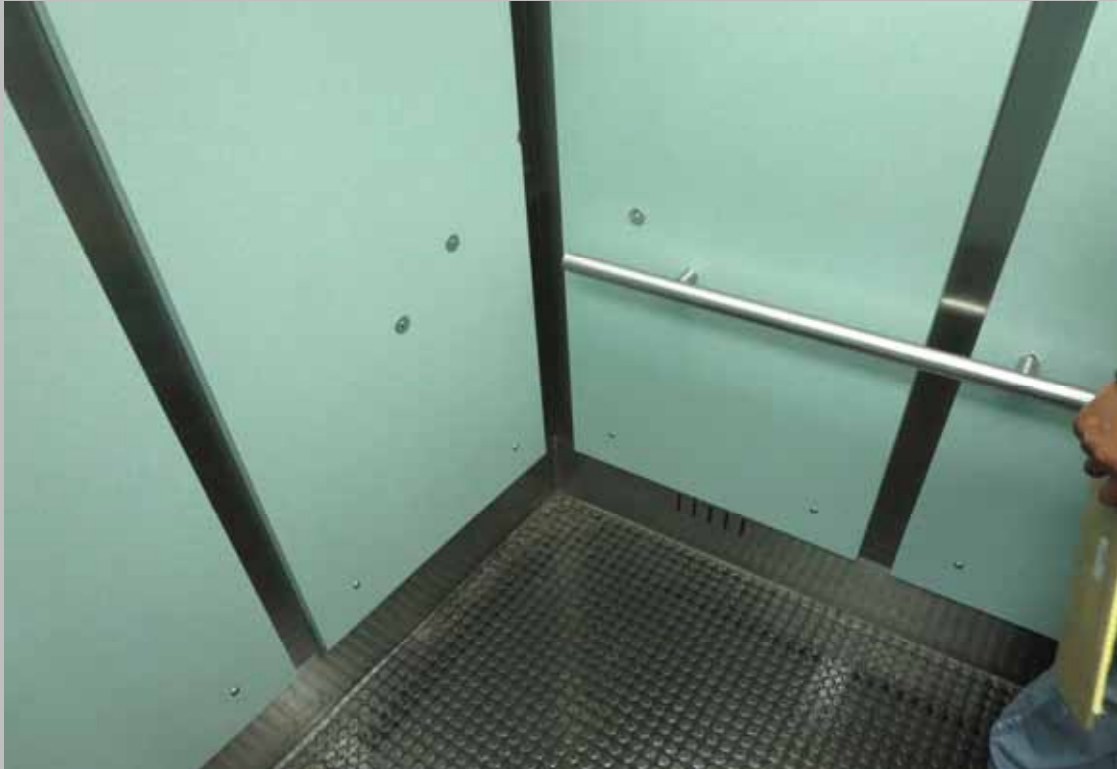
Refurbish interior elevator cabs (Non-Critical Repair)
