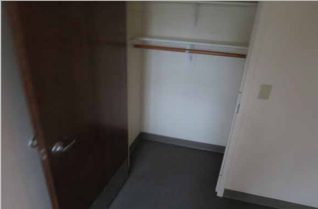
Replace dwelling unit carpeting (Non-Critical Repair)
