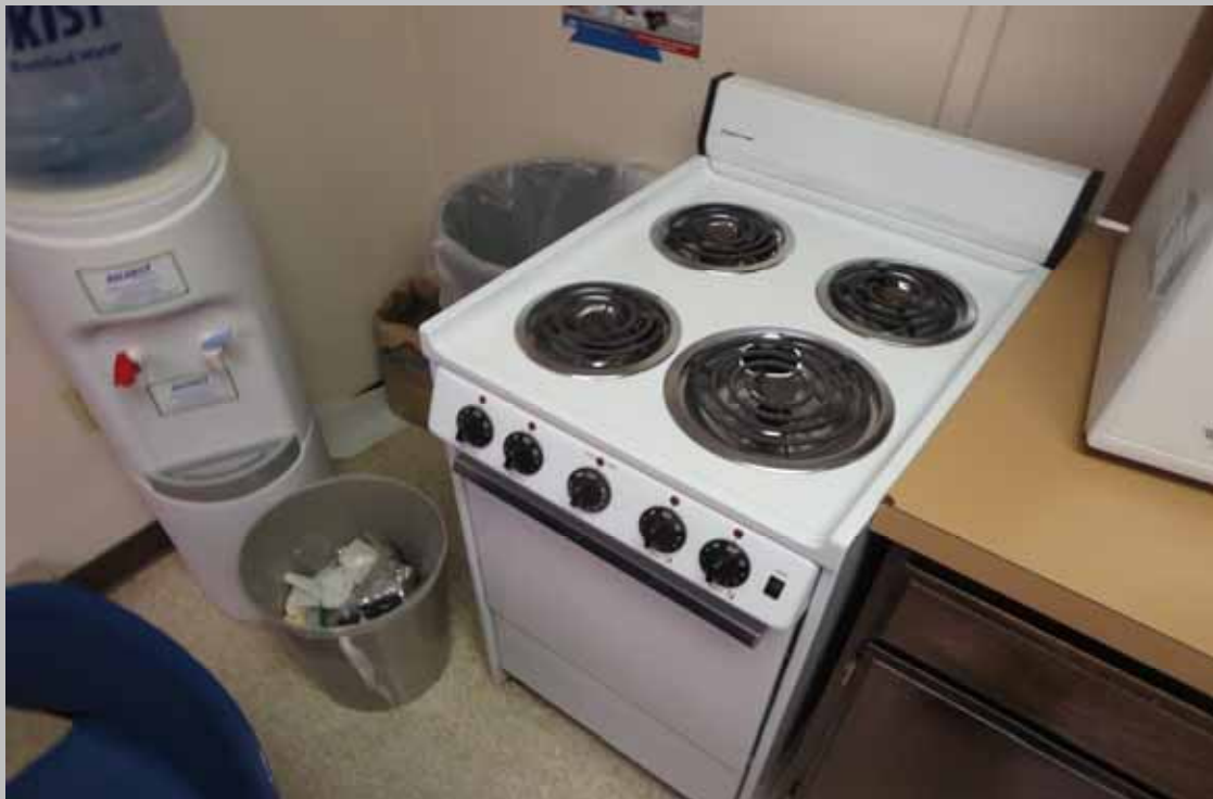
Replace ranges (Non-Critical Repair)
