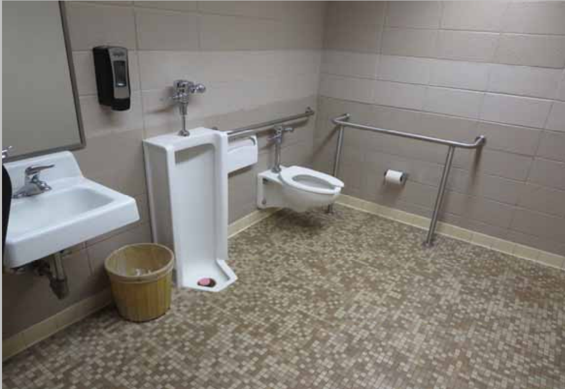
Replace common area restroom tile (Non-Critical Repair)
