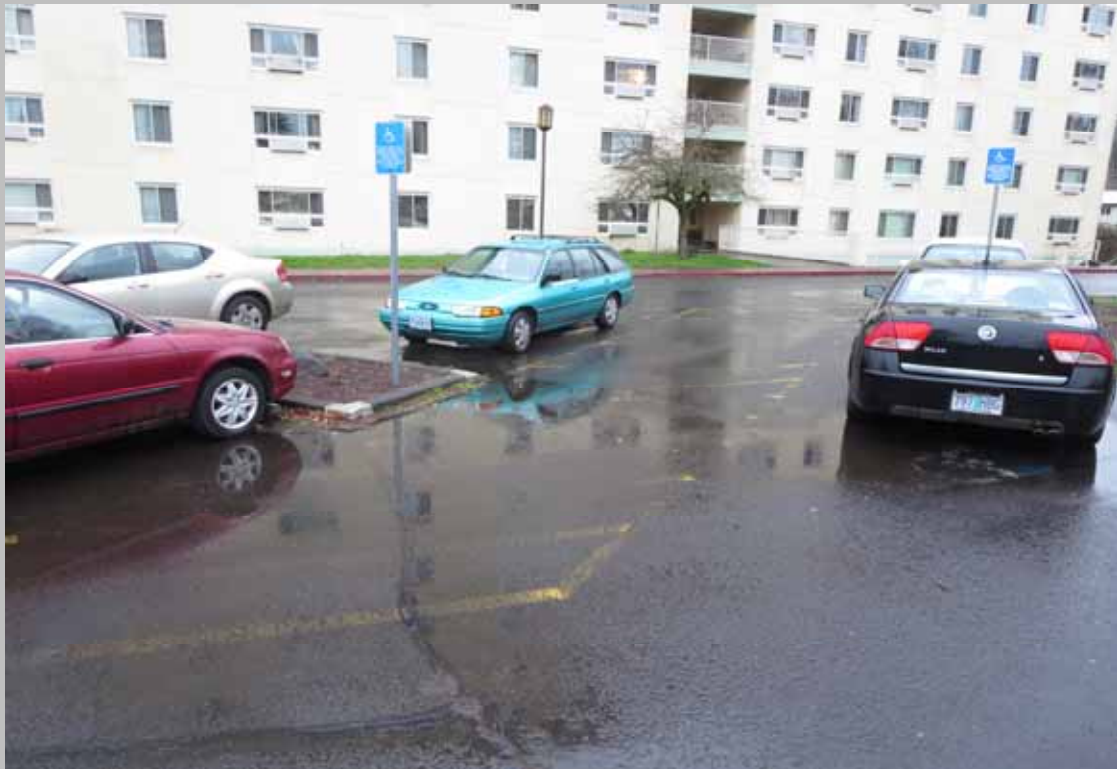
Restripe and configure handicapped parking spaces (Critical Repair)
