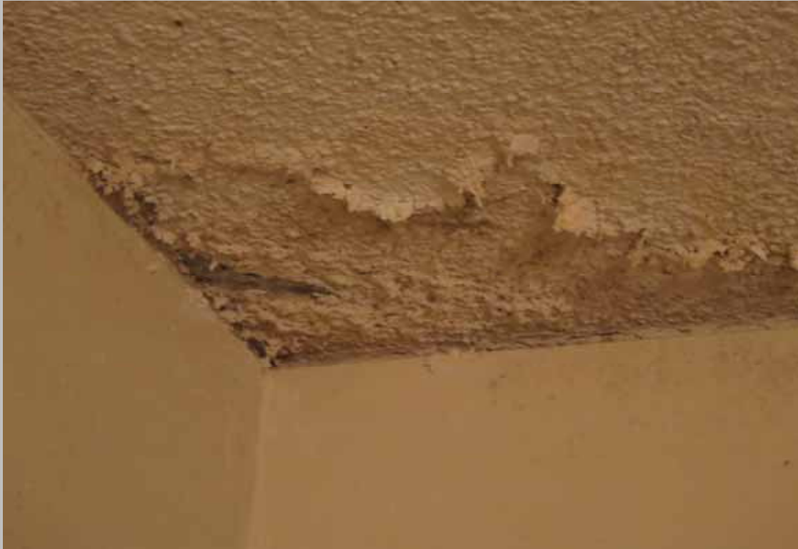
Repair ceiling at unit 306 (Non-Critical Repair)
