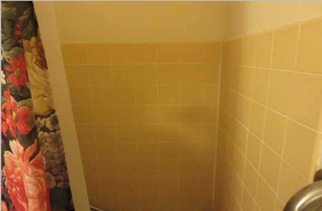
Replace tub/shower surrounds (Non-Critical Repair)
