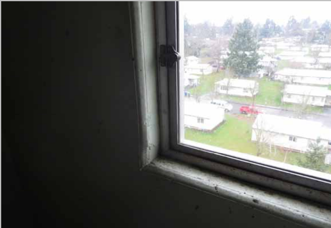
Replace original casement windows (Non-Critical Repair)
