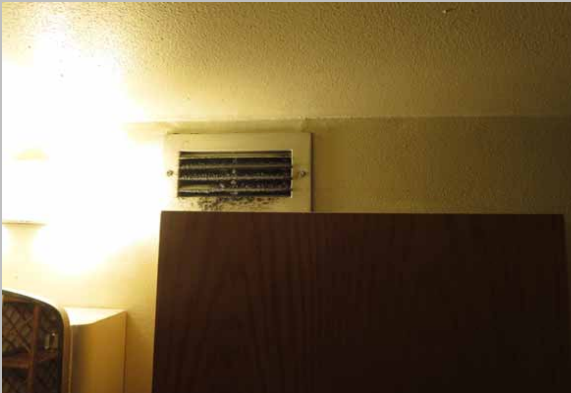
Clean dwelling unit ventilation ducts and registers (Non-Critical Repair)
