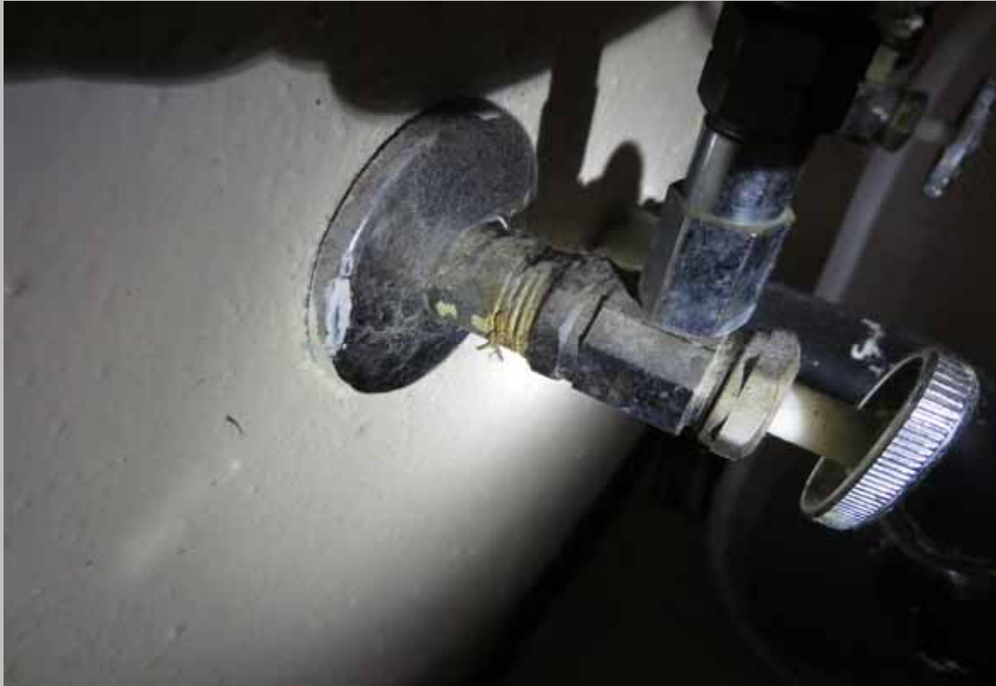
Replace original galvanized plumbing (Non-Critical Repair)
