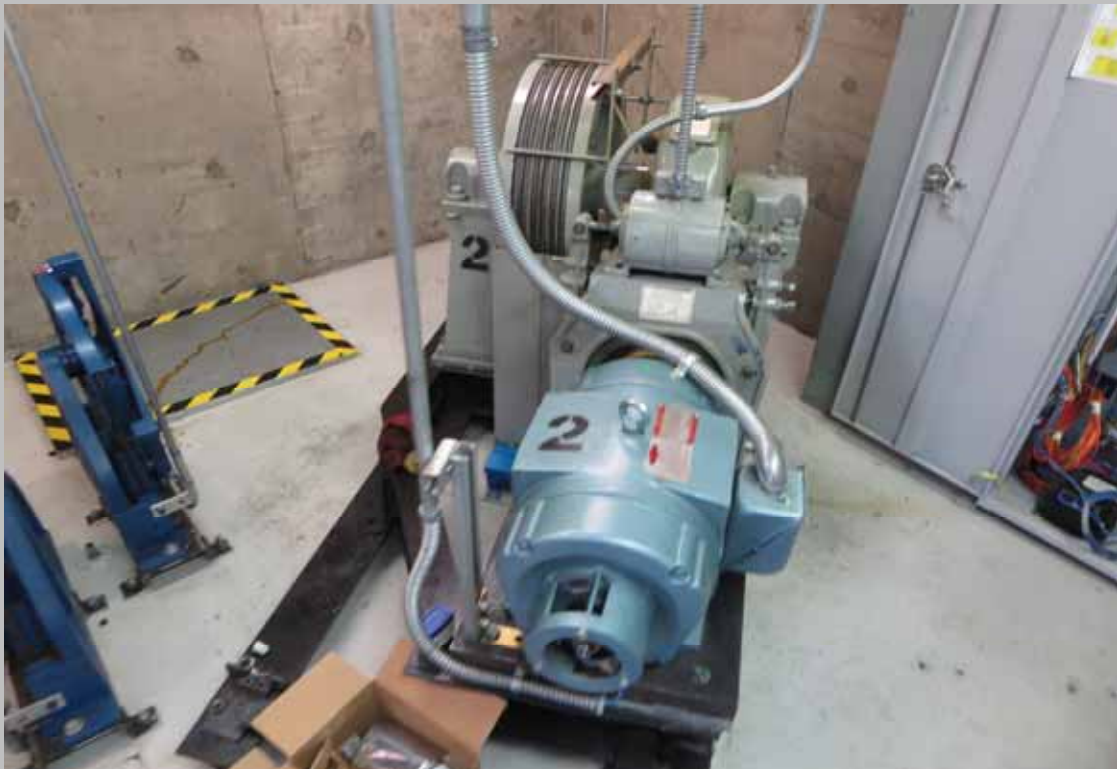
Replace elevator equipment (Non-Critical Repair)
