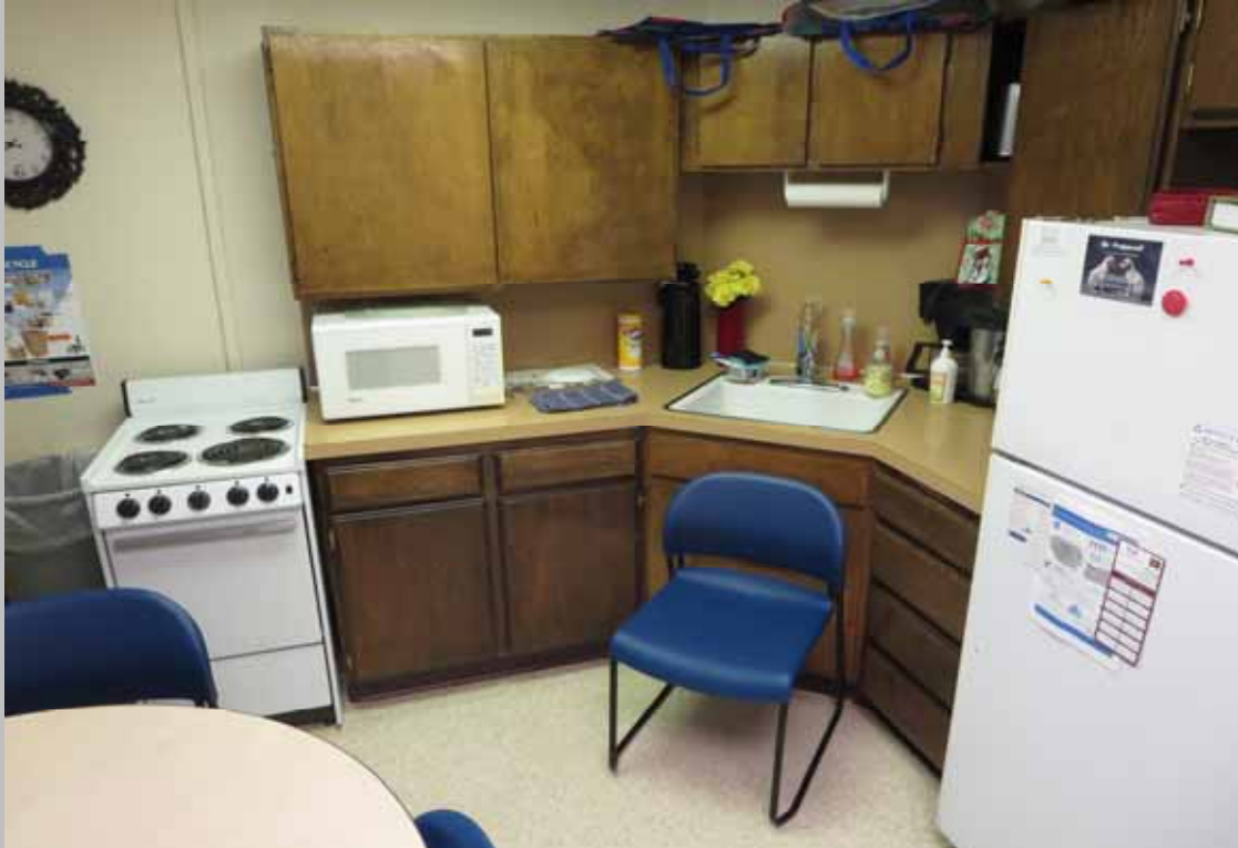
Replace common area appliances (Non-Critical Repair)
