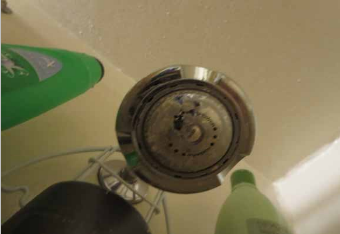
Replace showerheads with low-flow fixtures (Non-Critical Repair)
