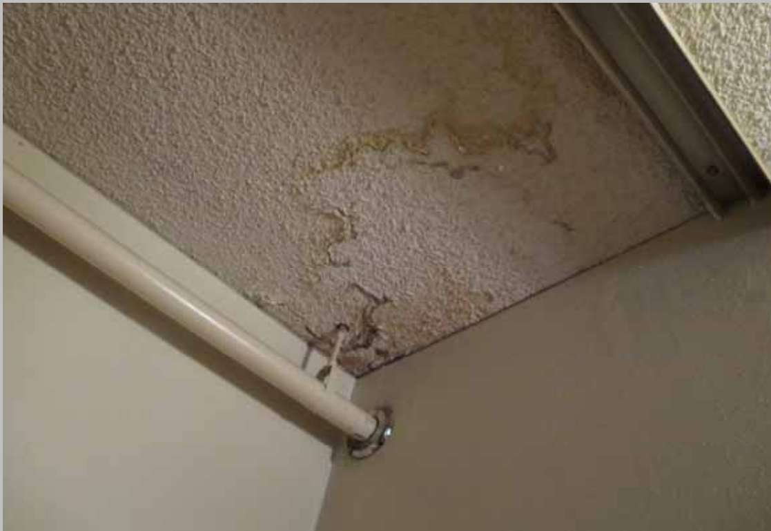
Repair ceiling at unit 304 (Non-Critical Repair)
