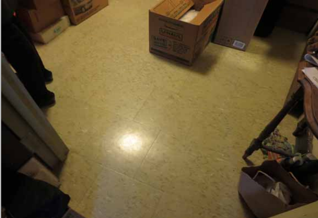
Replace dwelling unit VCT (Non-Critical Repair)
