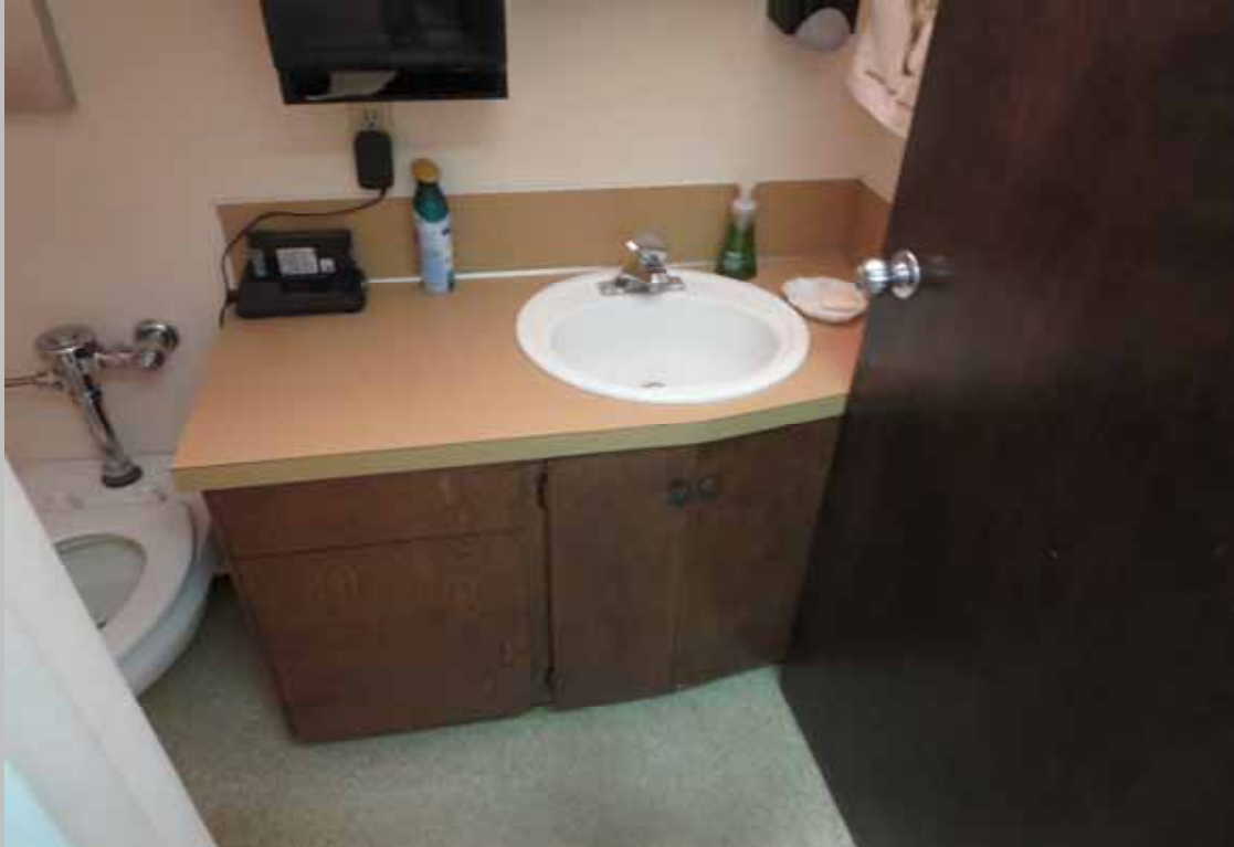
Replace common vanities (Non-Critical Repair)
