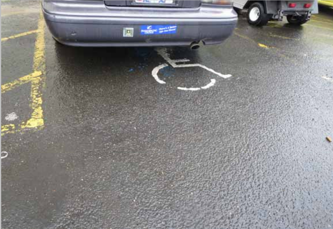
Restripe and mark parking areas (Non-Critical Repair)
