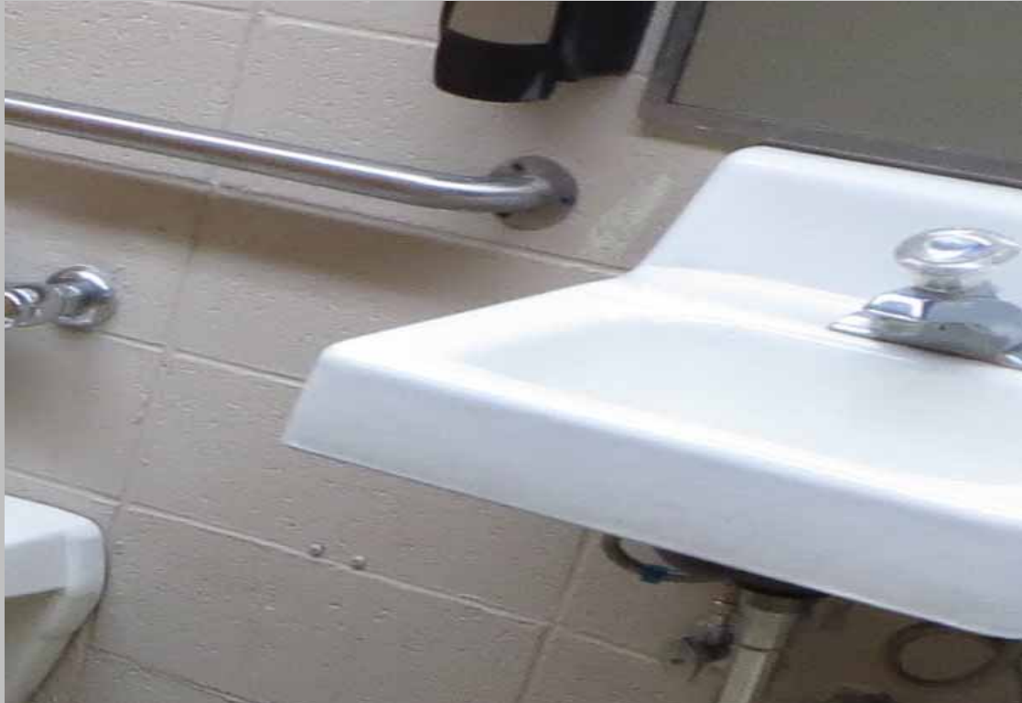
Install levered hardware at women's common restroom (Critical Repair)
