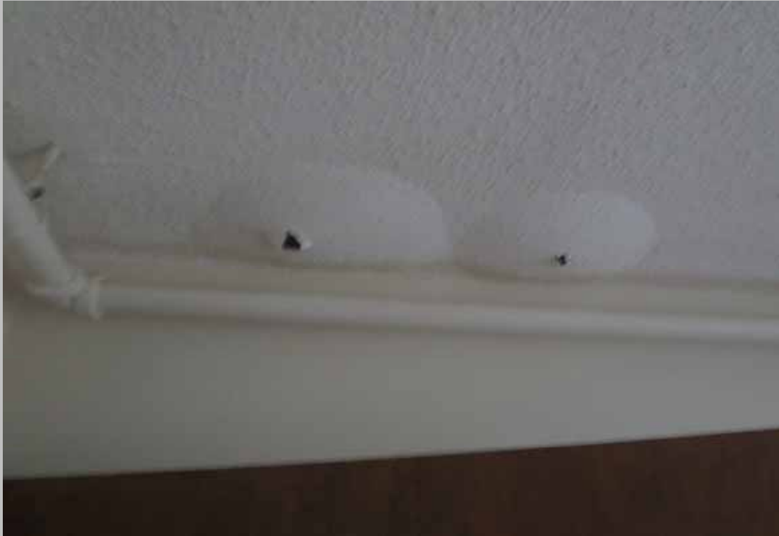
Repair ceiling at unit 711 (Non-Critical Repair)
