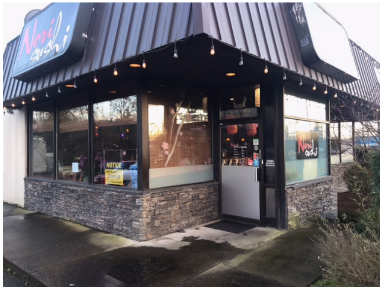
Main Front Door (Facing North) View 1
