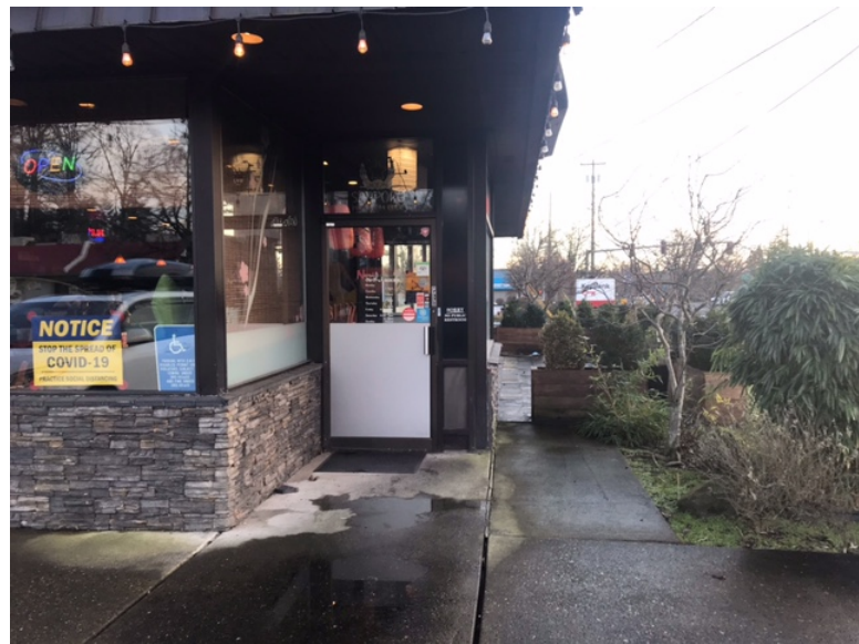
Main Front Door (Facing North) View 2
