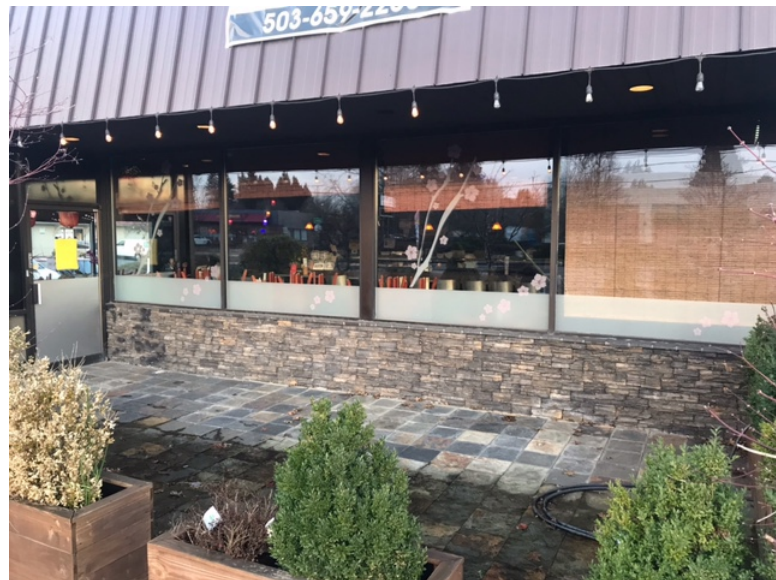
Outside Patio - View from 82nd Ave
