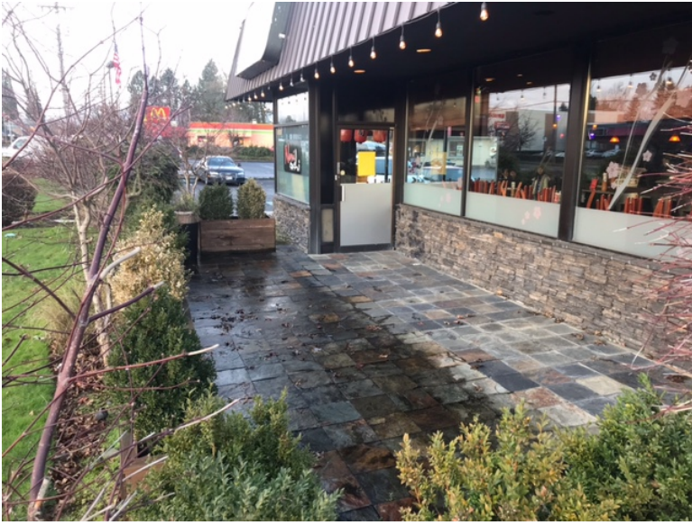
Outside Patio - South Door
