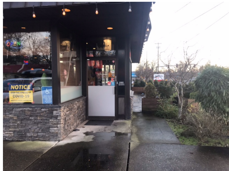
Main Front Door (Facing North) View 2
