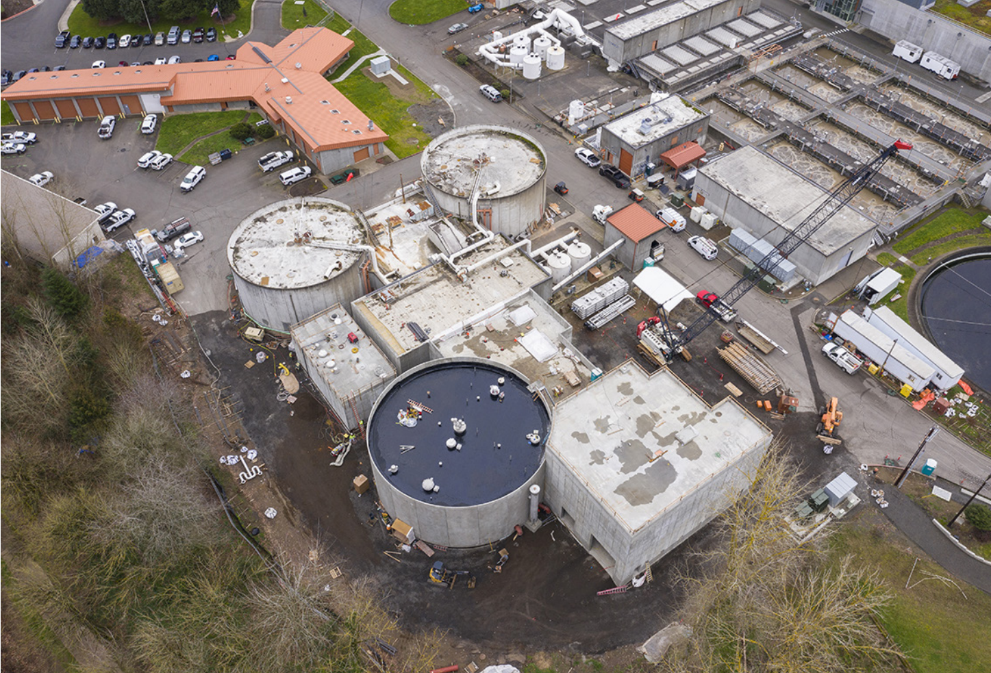
Progress on the Tri-City Solids Handling Improvement Project as of March 2020
