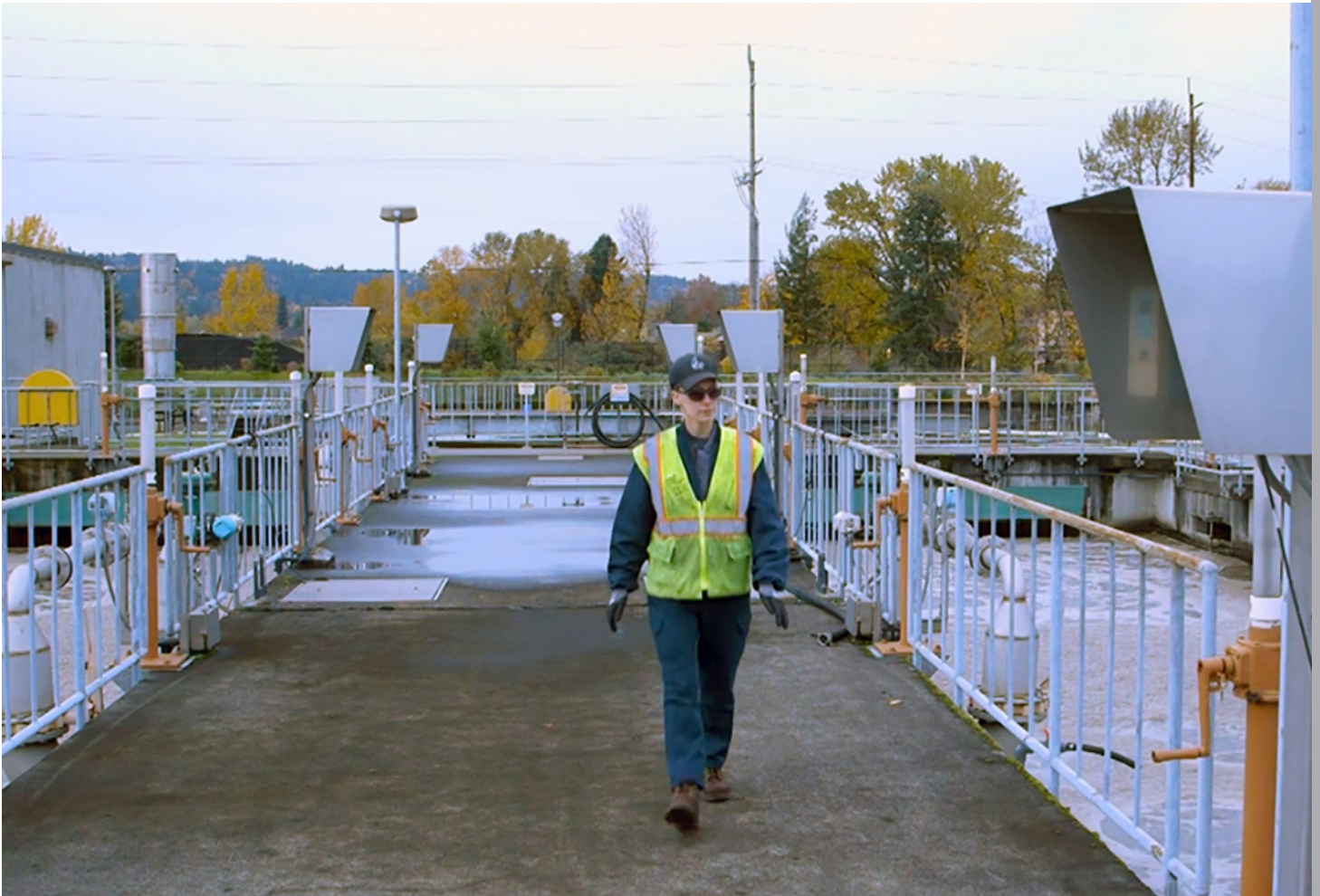
Tri-City Water Resource Recovery Facility
