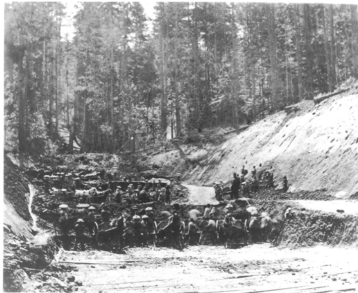
Chinese railroad workers working on the O&C railroad, south of Portland. Oregon Historical Society, Folder 238-A.
