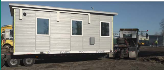
Construction of Clackamas Village
