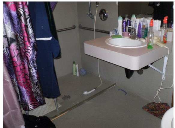
Photo #30: Typical accessible shower
