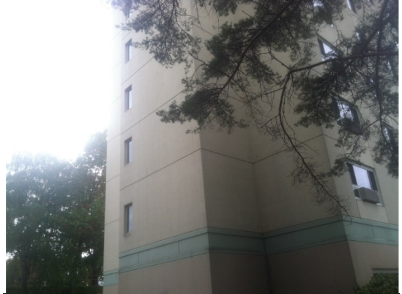
Photo #8: East elevation
