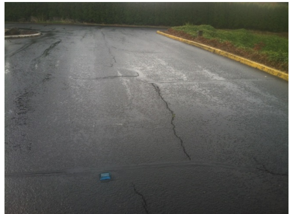
Photo #52: Asphalt paving
