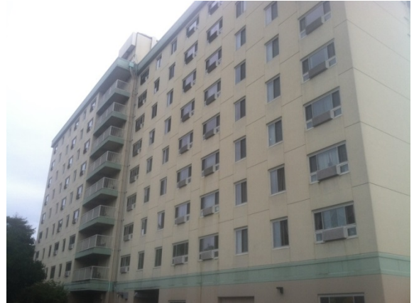
Photo #2: North elevation
