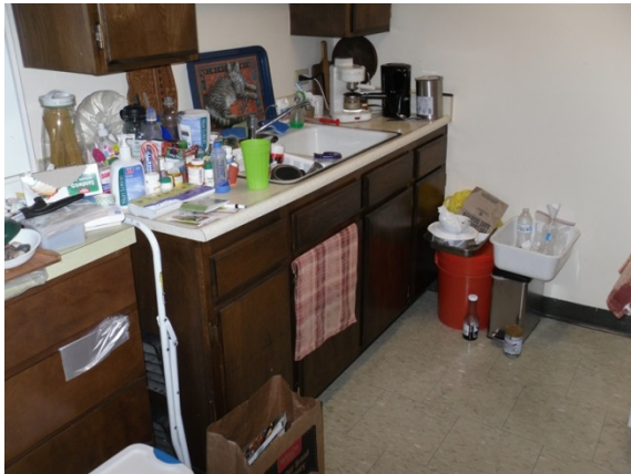
Photo #21: Typical kitchen cabinets
