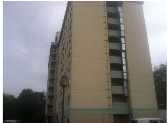
Photo #4: West elevation
