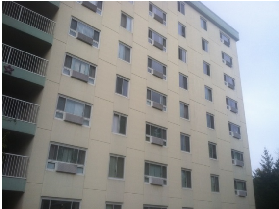
Photo #3: South elevation
