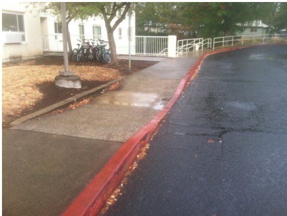
Photo #51: Accessible sidewalk
