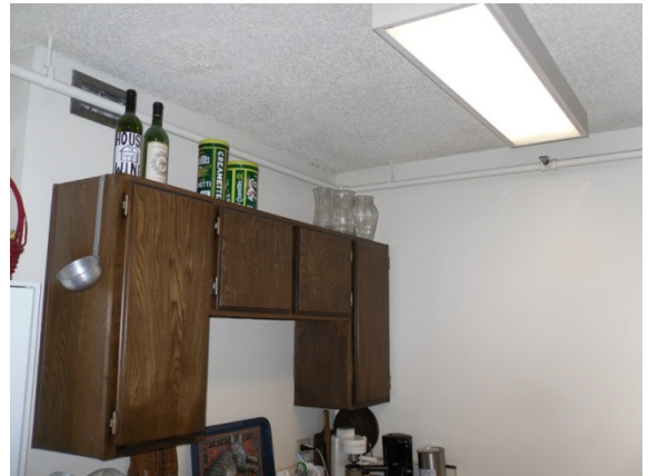
Photo #22: Typical kitchen finishes
