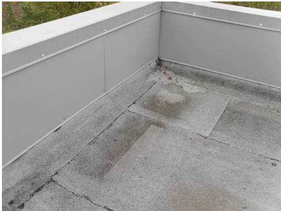
Photo #11: Roof finishes
