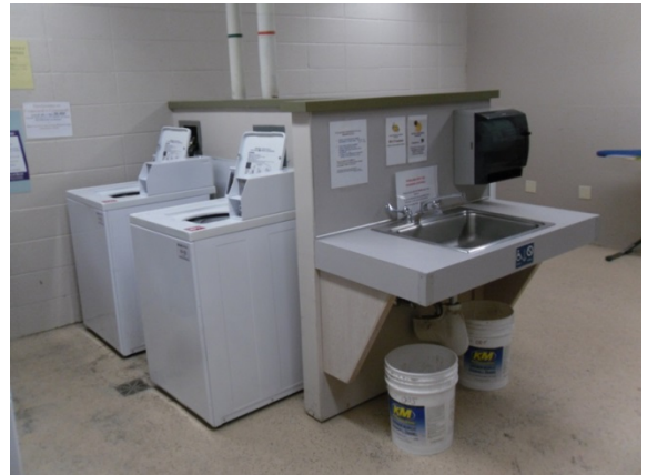
Photo #18: Laundry room
