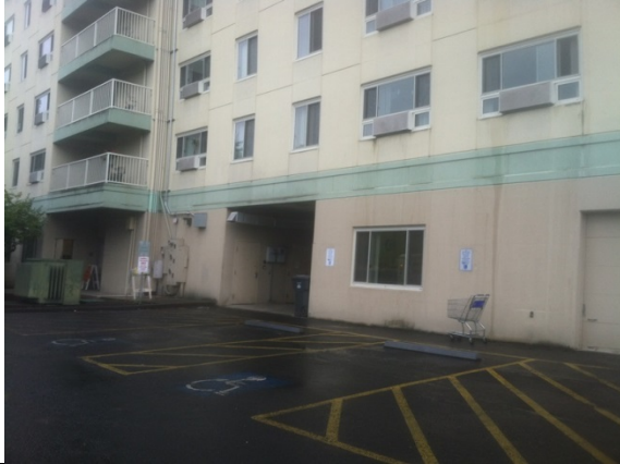
Photo #7: North elevation
