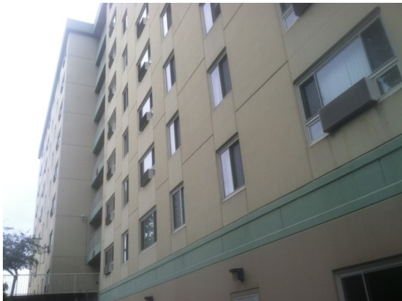
Photo #5: South elevation
