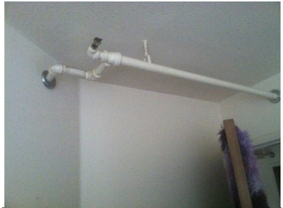
Photo #26: Typical apartment finishes
