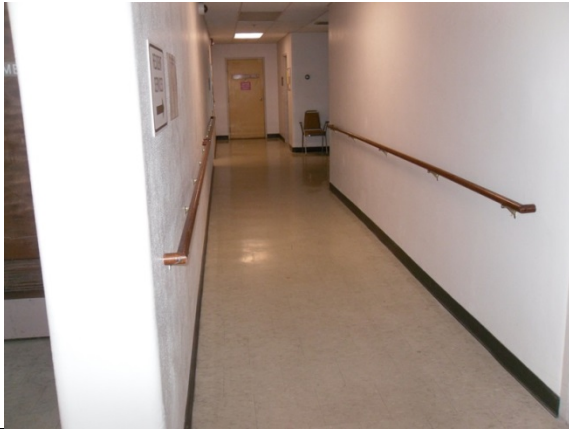
Photo #13: Typical corridor
