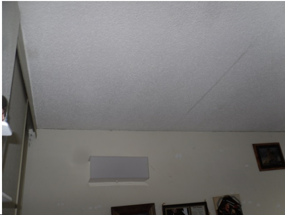
Photo #25: Typical apartment finishes
