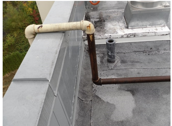
Photo #12: Roof finishes
