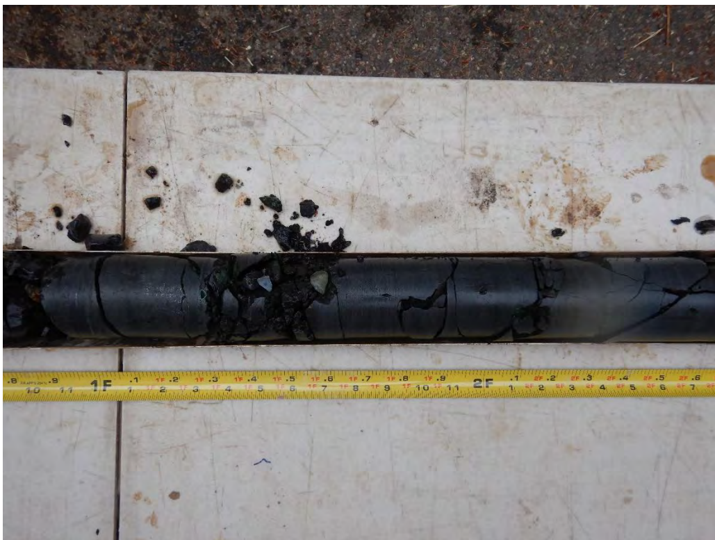
B: Boring LT-2, Sample R-2, Depth 33.0-36.0 ft. Image 2 of 3.
