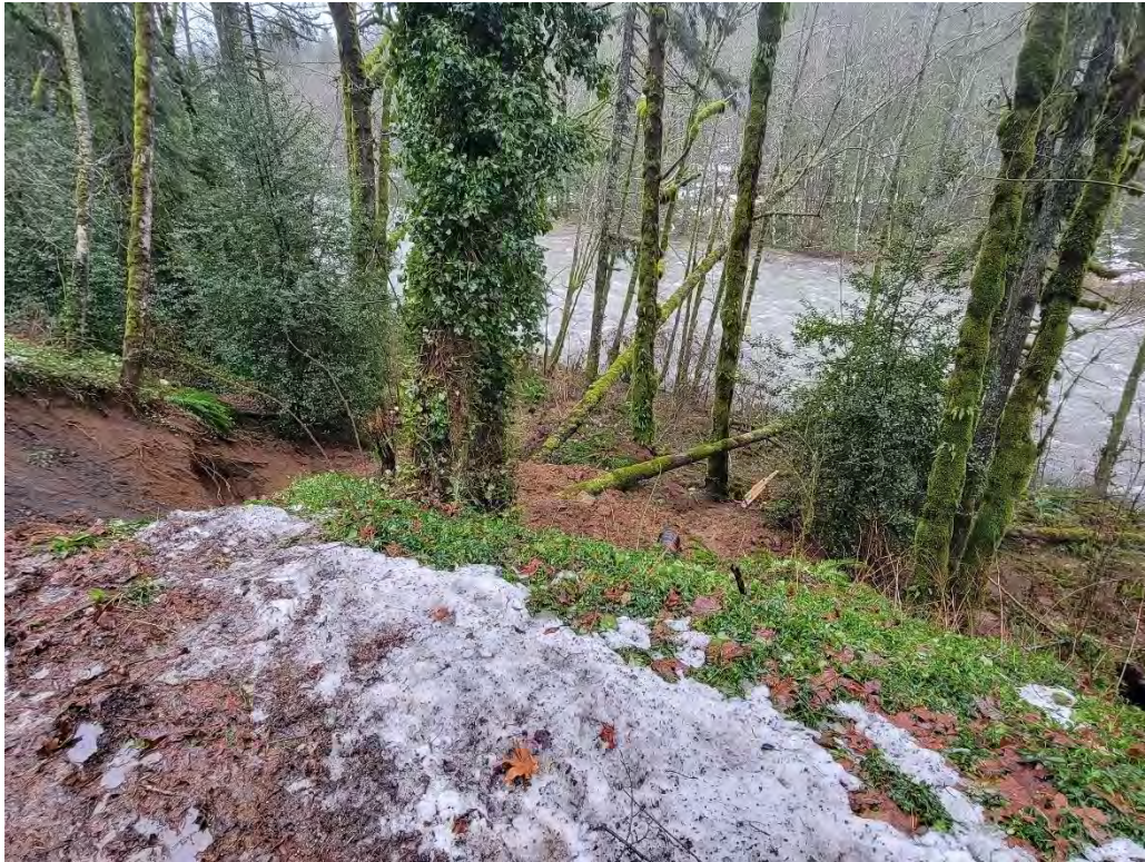
A: View looking southeast at toe of landslide, above the Sandy River. (East Barlow Trail Road)
