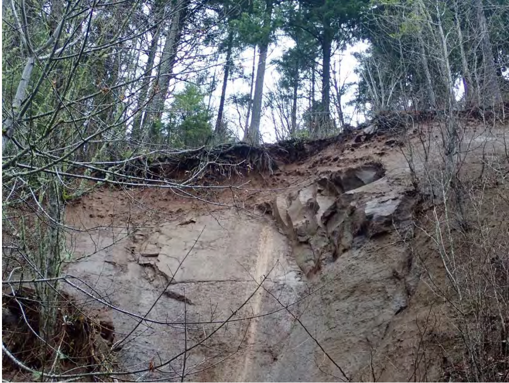
A: View looking north at crest of slope, undermined hazard trees, and potential rockfall area. (SE Bull Run Road near SE Laughing Water Road)
