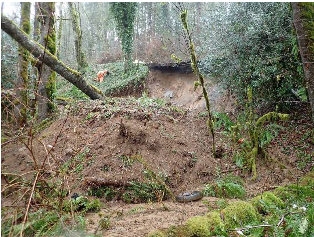
B: View looking northwest at landslide toe, undermined road, and blocked drain near person. (East Barlow Trail Road)
