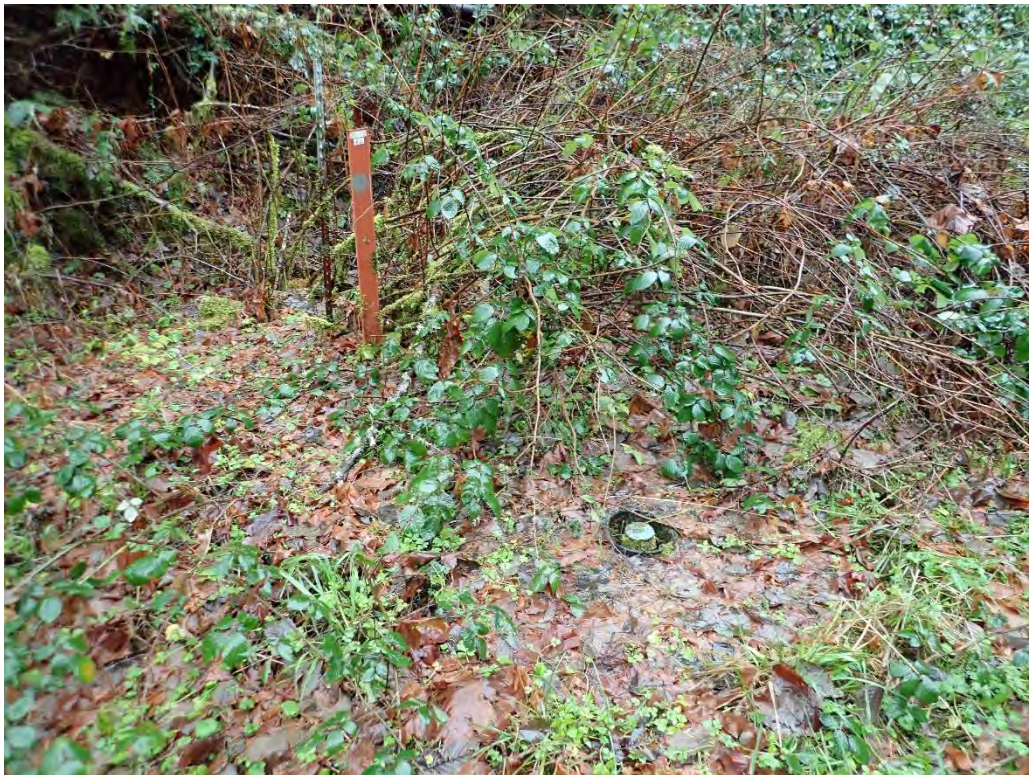
B: View of existing geotechnical instrumentation installed. (SE Bull Run Road between SE Ten Eyck and SE Phelps Roads)
