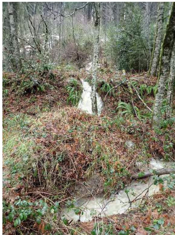
B: View of discharge from settlement pond in quarry into unlined ditch. (East Barlow Trail Road)
