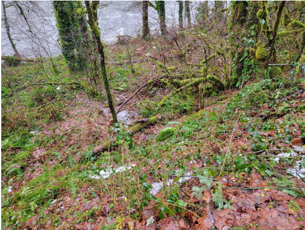
A: View looking south at culvert discharge, east of the landslide. (East Barlow Trail Road)
