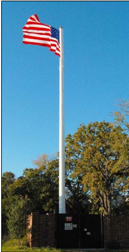
Figure 24: There are antennas in this flagpole.
