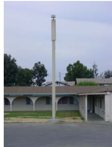
Figure 25: A parking lot light with an antenna shroud that complements the pole.
