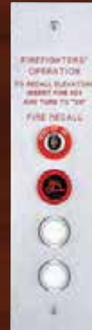
Intermediate hall station With fire services devices
