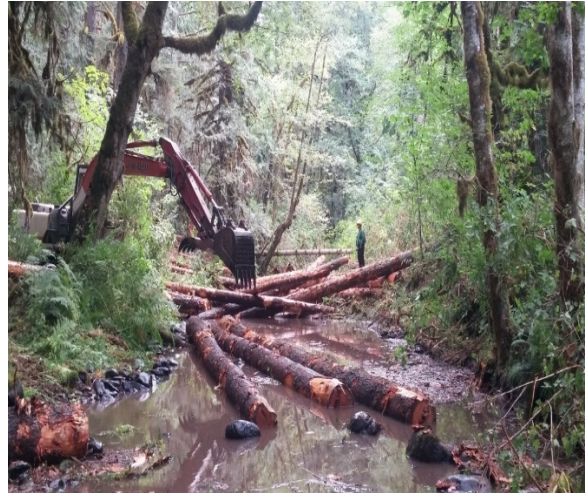
Log placement in Smith Creek.
