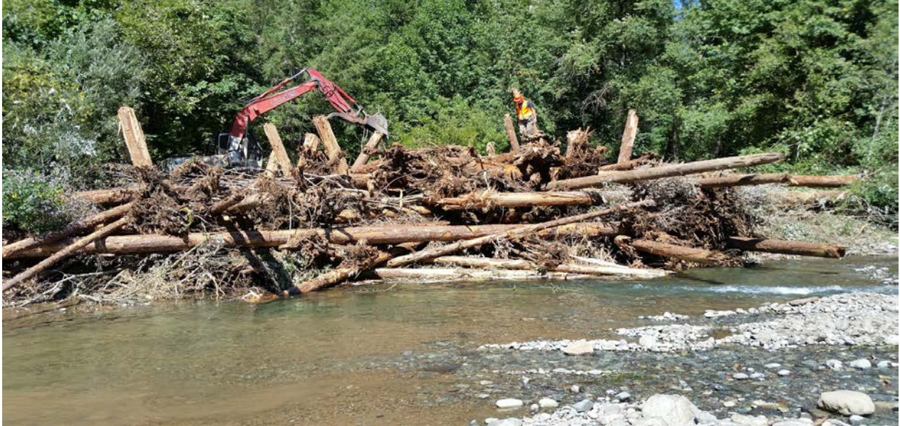
Fish habitat structure during construction.
