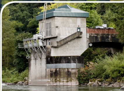
Drinking Water Intake Facility
