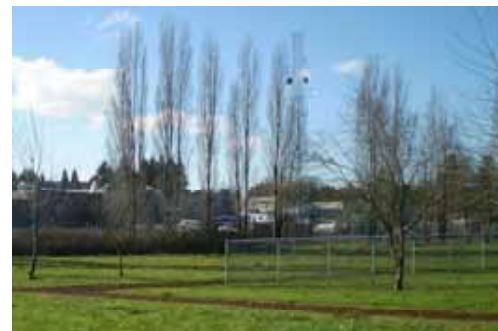
Type G Fence foreground, Storage Building Type D Fence background, Adult Detention Facility
