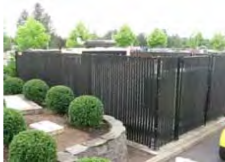
Type H Fence, Public Services Building
