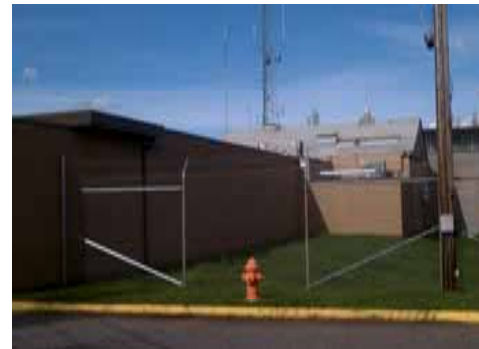
Type C Fence, Adult Detention Facility
