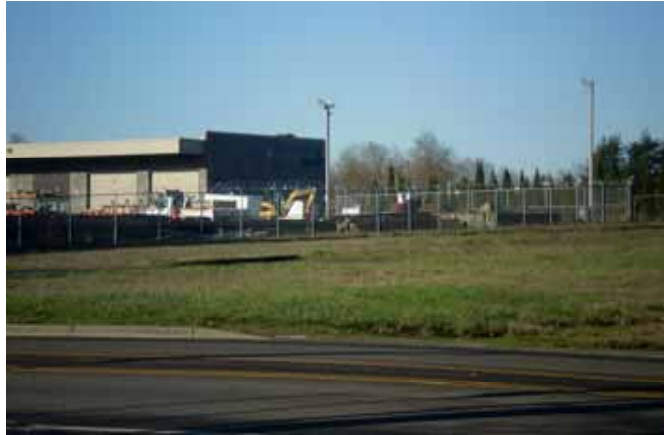
Facility Enclosure at PGE on Warner Milne Road
