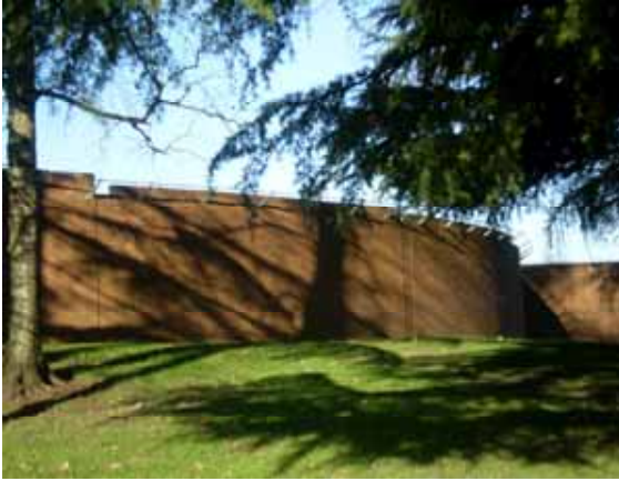
Facility Enclosure at PGE on Warner Milne Road
