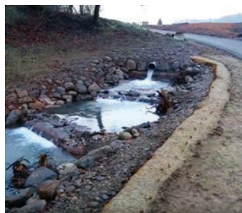
Stormwater funneled to the site
