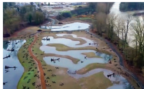
Aerial view of the 15-acre Carli Creek Water Quality Facility
