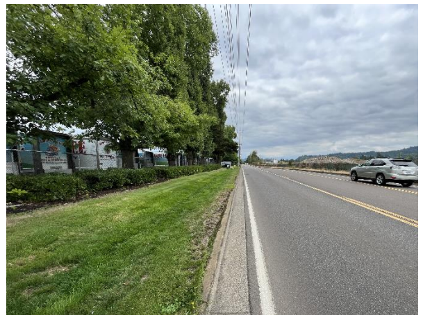
Figure 28: Example of Missing Sidewalks in Study Area
