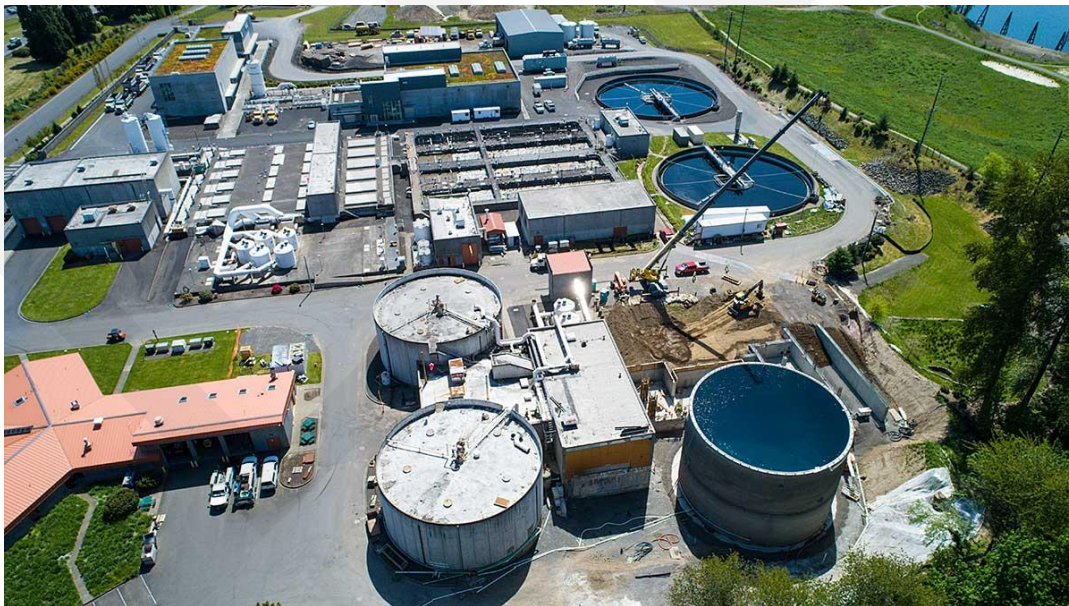
Figure 25: Environmental Monitoring example
