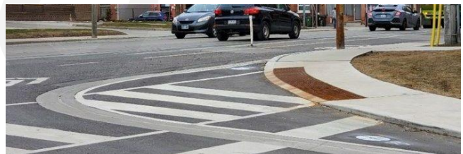
Figure 35: Truck Apron at Intersection Example
