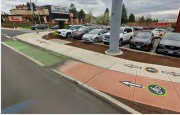
Figure 33: Bicycle and Pedestrian Ramp Examples
