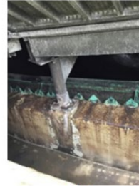
Picture 8. Primary Basin 2
