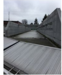
Picture 9. Primary Basin 1
