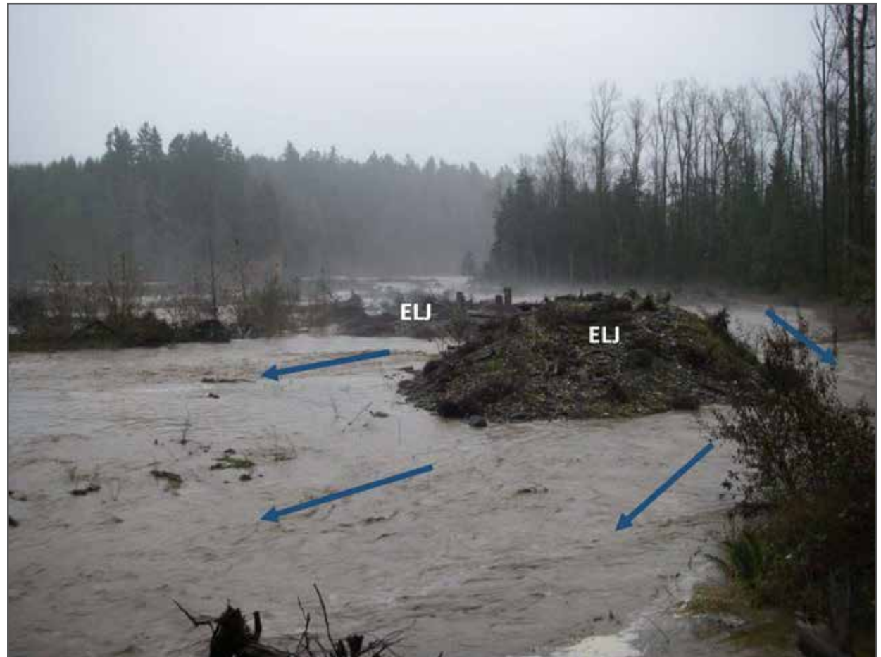
Figure 23. The Upper Puyallup project during high flow in 2014 looking upstream at two of engineered logjams (ELJs) in the energy dissipation area (side channel zone). View is from complex large wood revetment on Upper Puyallup River's left bank. The ELJs are splitting flow into smaller channels before the flow reaches the bank. The ELJ is one of six forming an array of structures to keep the main channel from approaching the bank. Photo by Tom Nelson.
