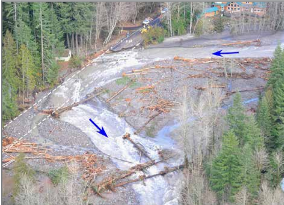
Figure 12. Along a road washout in the Upper Sandy River after the 2011 flood, large wood scattered and lodged along the river, increasing roughness and complexity of the channel. Historic confinement and clearing of the river has prevented the river from spreading out and dissipating its erosive energy. The more space the river has, the lower the river's erosive power. Allowing the river space to move and connect broader floodplains not only reduces flood risk, but expands salmon habitat. Photo by PGE
