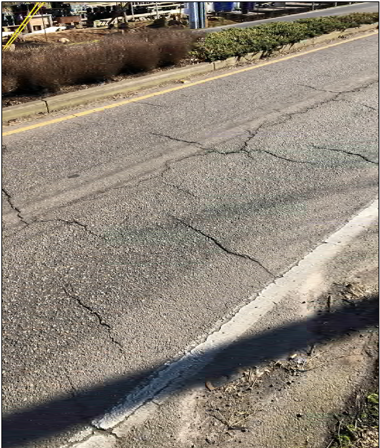
There are moderate severity non-wheel path longitudinal and transverse cracks, and some are interconnected showing patterns of onset of block cracking.
