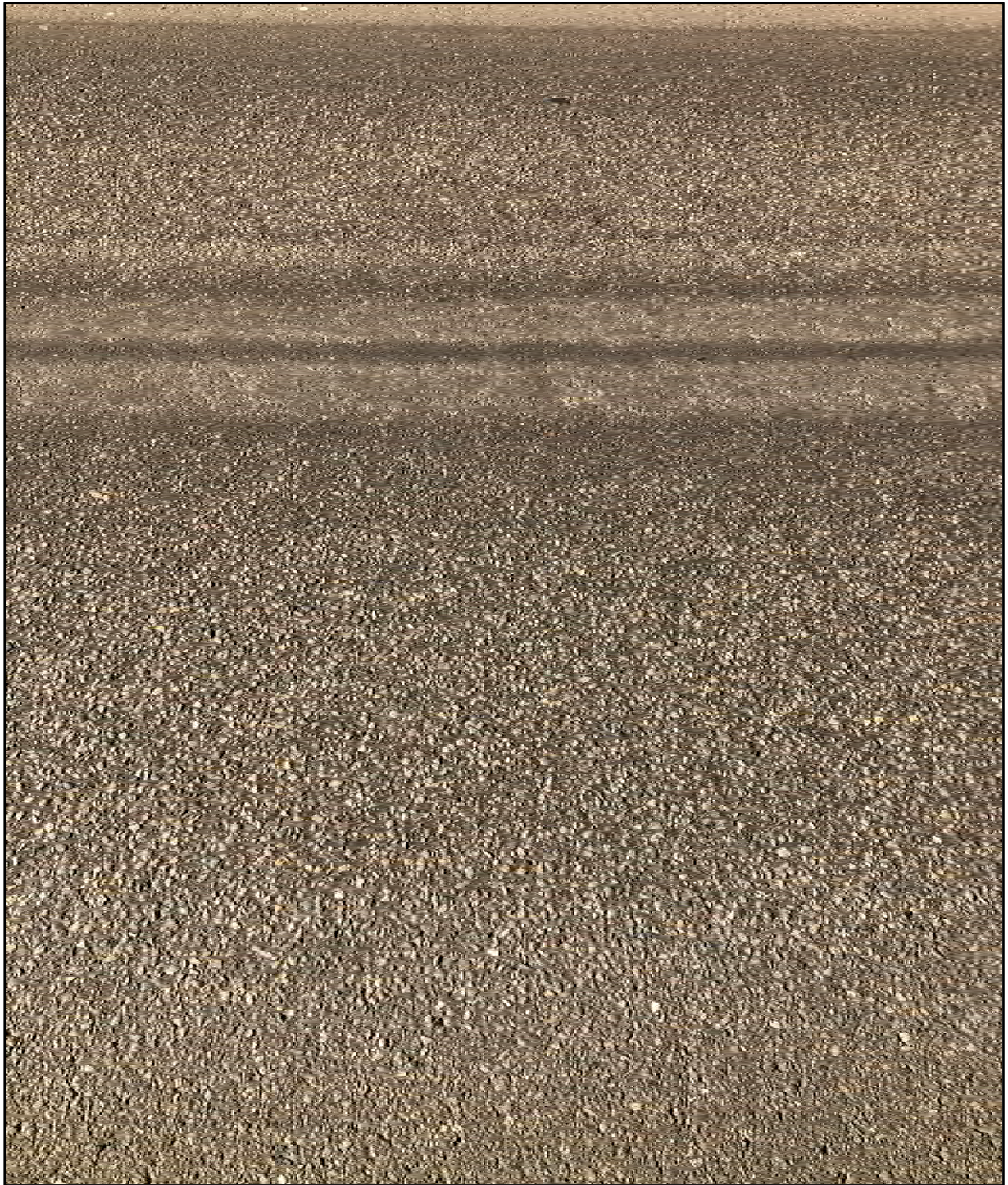
This section shows moderate severity raveling especially in the wheel paths.
