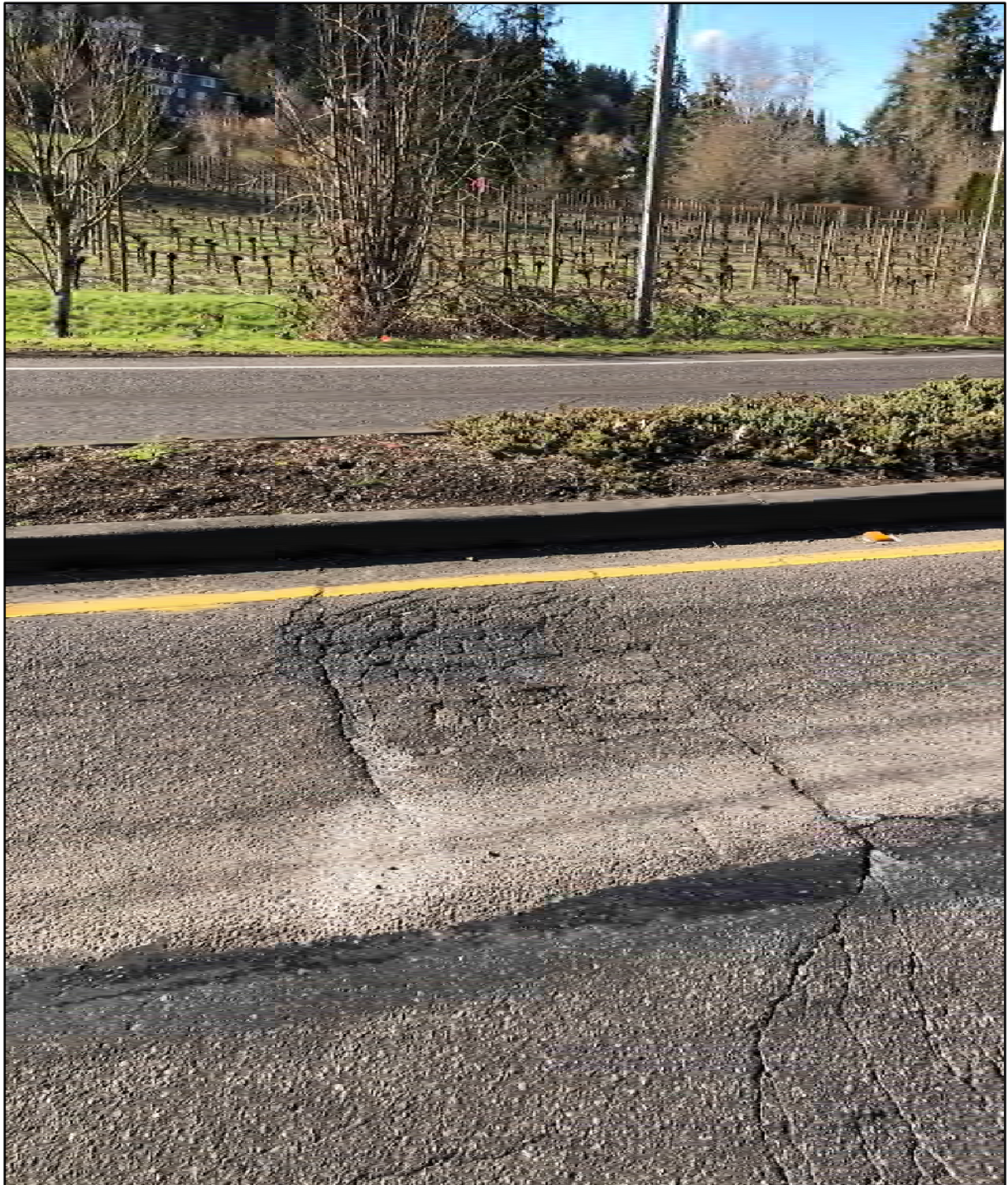
There is a small area (4' by 4') exhibiting high severity fatigue cracking at station 1+15.
