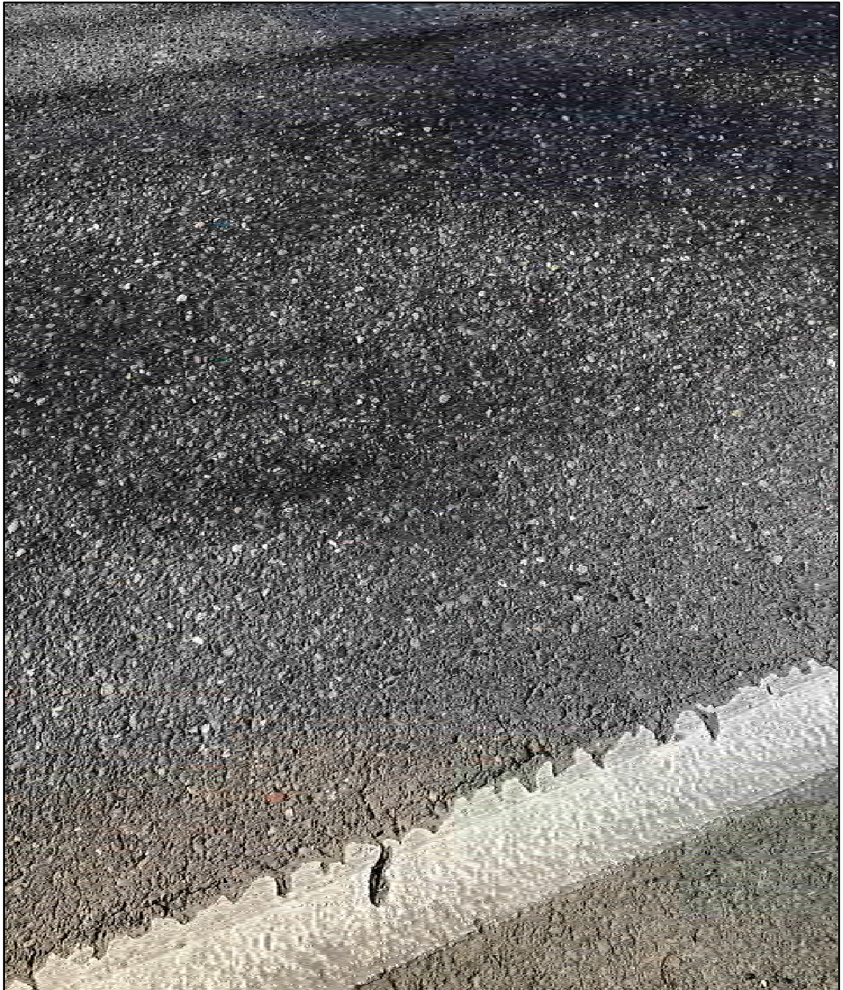
This section exhibits moderate severity raveling especially in the wheel paths.
