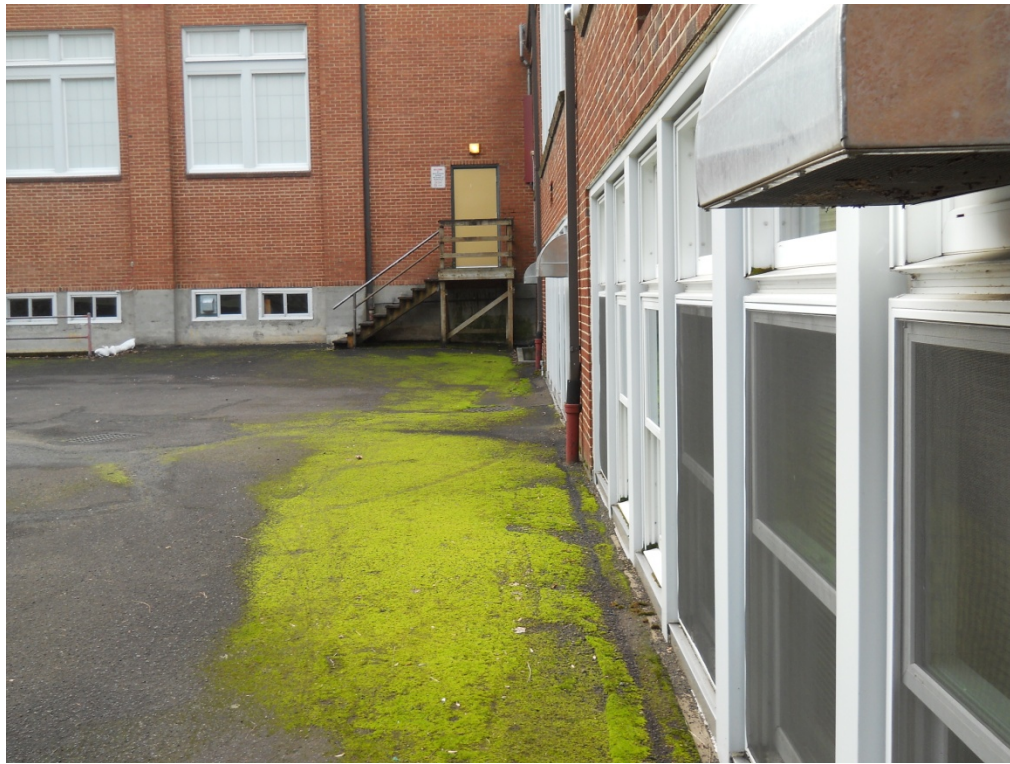
PHOTO 5: Looking west-southwest along the addition
