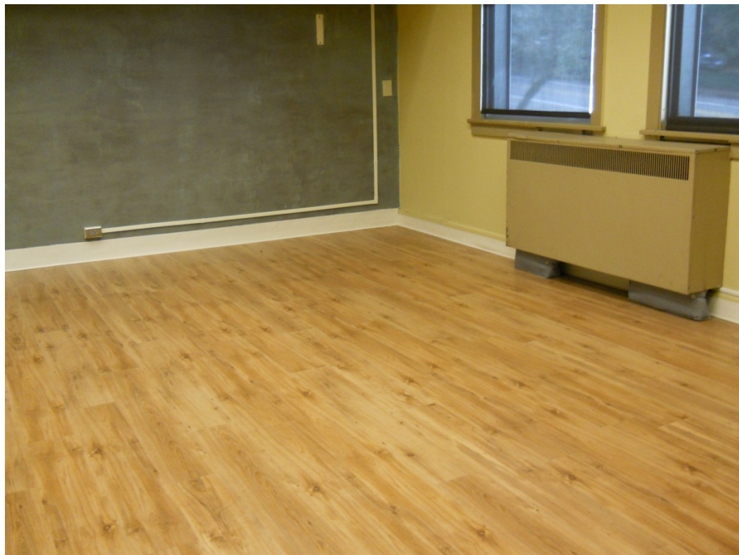
PHOTO 26: Staff room located on upper level, recently refinished
