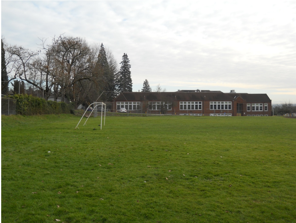
PHOTO 11: North side of school looking southeast across the field
