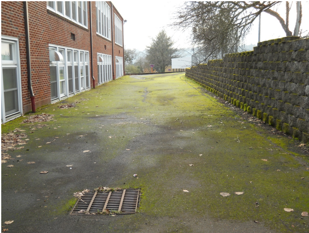
PHOTO 4: North side of school looking west-southwest
