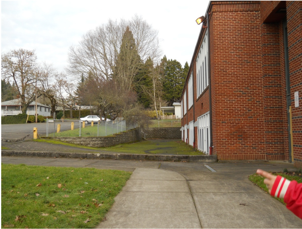
PHOTO 3: North side of school looking east-northeast along the addition to the original building
