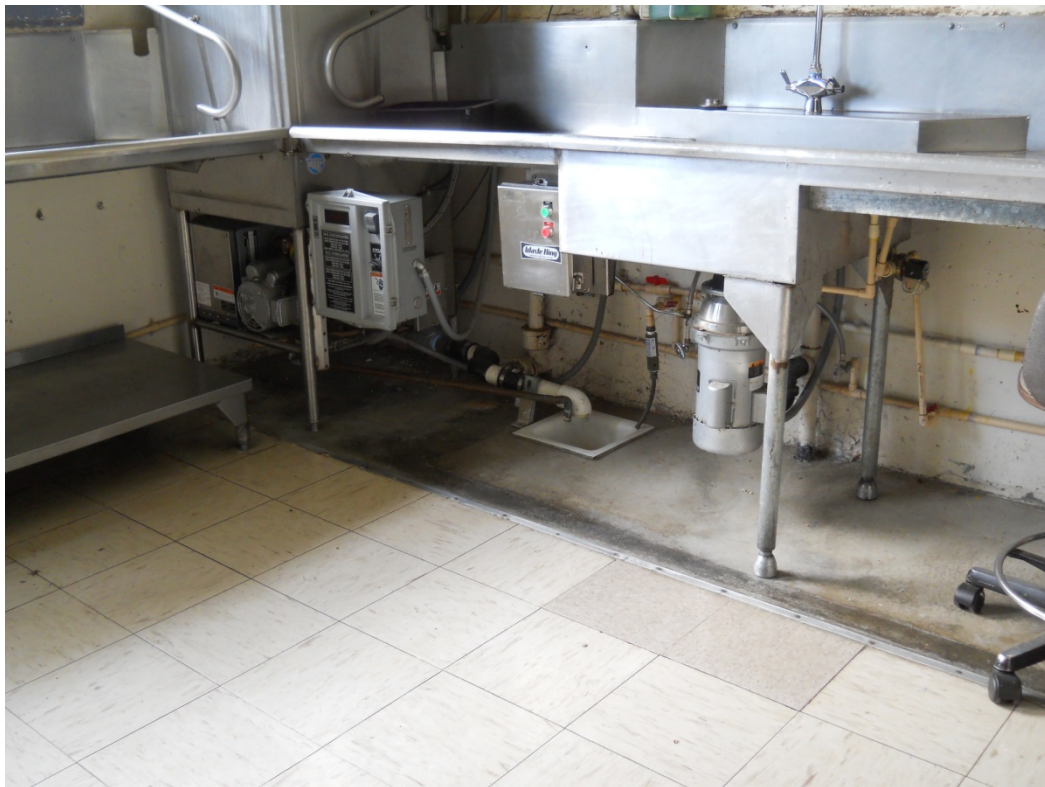
PHOTO 18: Kitchen area located on the lower level
