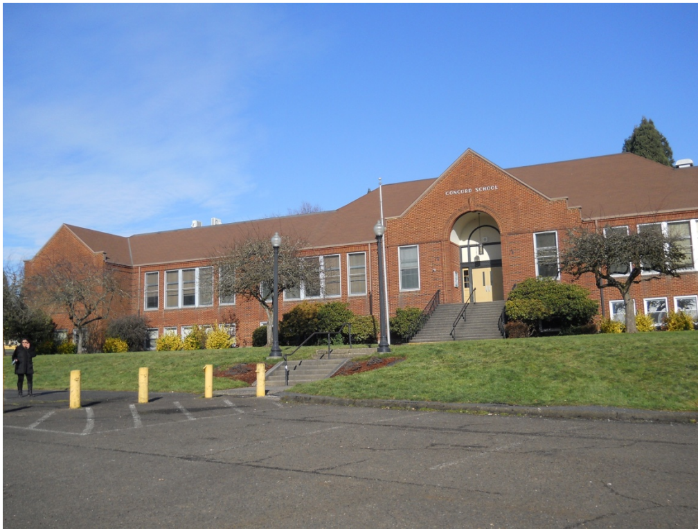
PHOTO 1: West side of school looking north from parking lot
