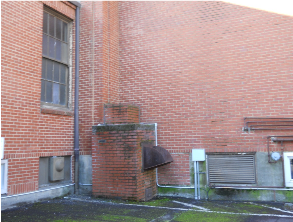
PHOTO 7: Former incinerator located on the east side of the school
