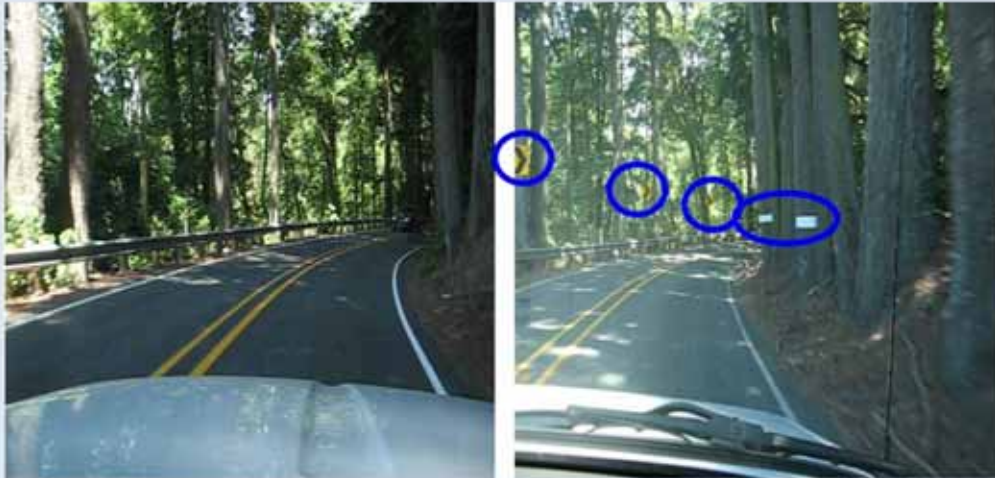
Chevron Signs and Reflective Markings Improve Visibility on Wilsonville Road
