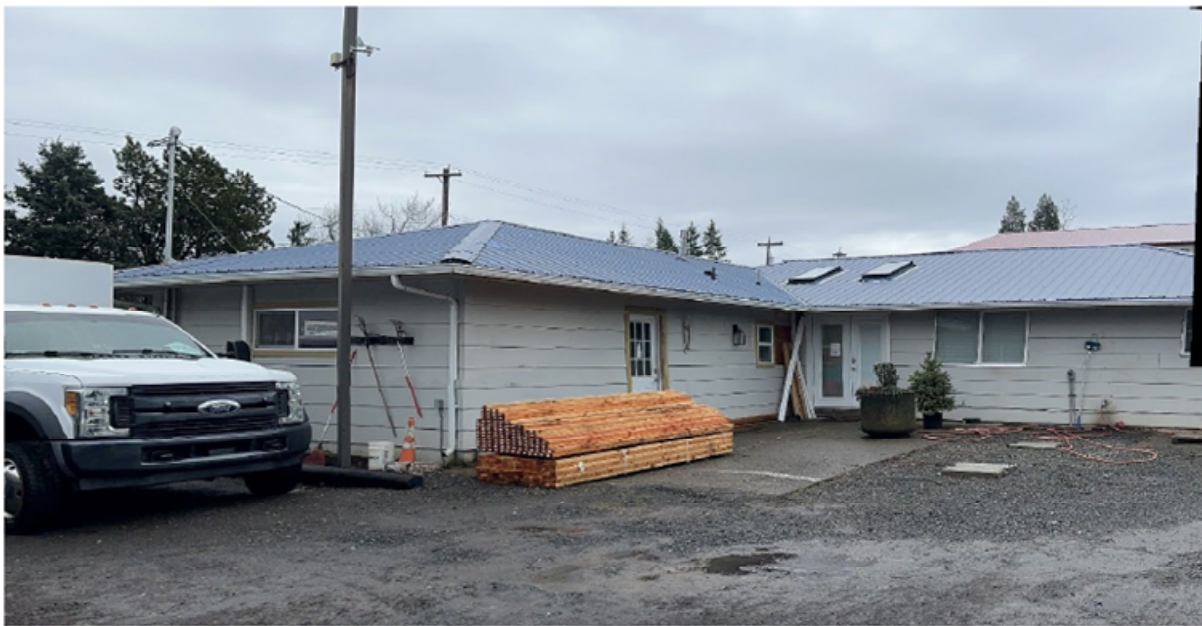
Figure 7. North-facing façade of existing structure
