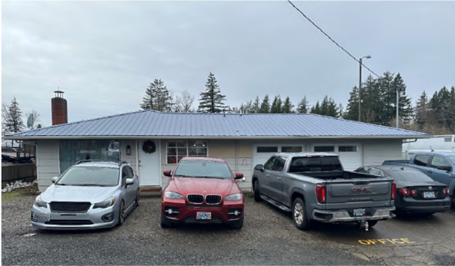
Figure 6. Front, or east-facing, façade of existing structure
