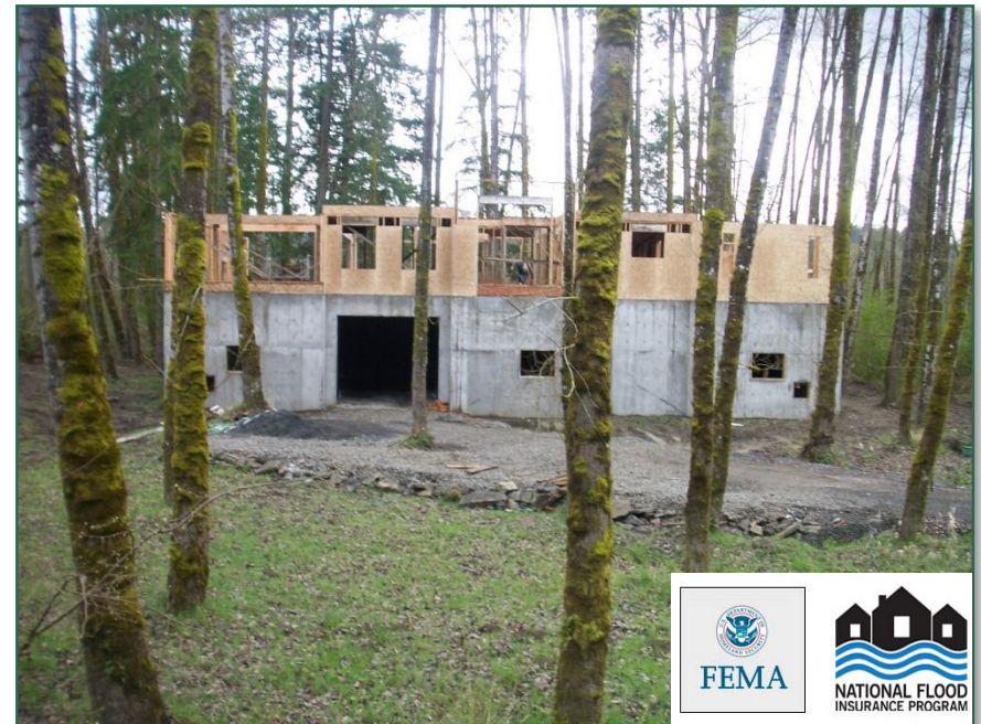
Above: Elevated home under construction in floodplain of Clackamas River.
