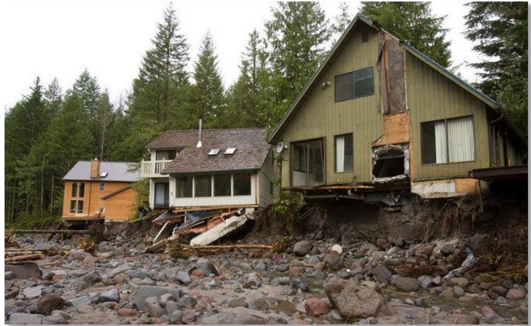
Above: Three damaged homes in a row from 2011 Sandy River flooding.
