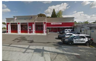
Gladstone Fire Station
