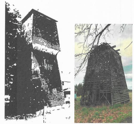
*Water Tower (rear view) showing the missing third floor which once stored water and housed a windmill-driven pump, today a hollow decrepit shell.*
