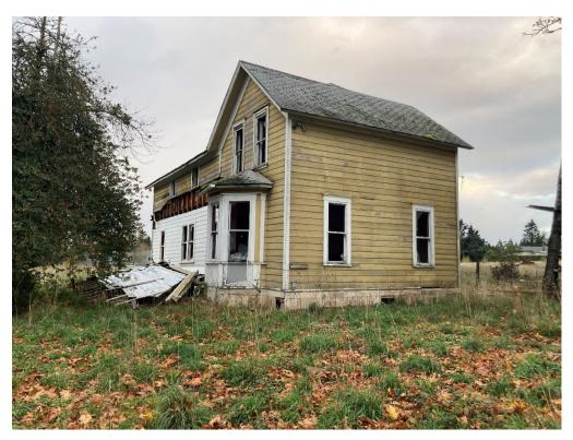
*House today (showing broken windows, exposed foundation and collapsed porch blocking the front door)*
