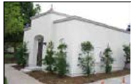
Figure 6: Equipment is concealed within this enclosure with the air conditioning units located on the roof behind the parapet.
