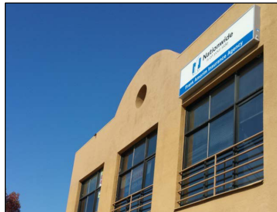
Figure 13: Antennas are concealed behind the circular element.
