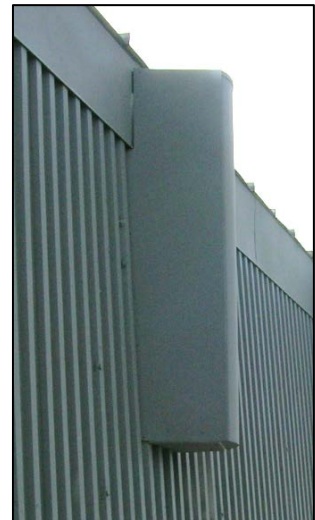
Figure 17: Antenna skirts and chin straps used to conceal mounts and cables.
