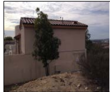
Figure 5: The generator is concealed inside the building above the existing equipment enclosure.
