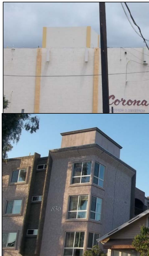
Figure 28: Two rooftop boxes that replicate existing building elements well.
