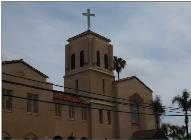
Figure 14: Façade-mounted antennas with antenna skirts and chin straps, placed symmetrically and painted to match.
