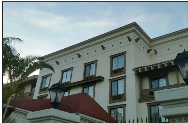
Figure 4: A completely concealed WCF. There are antennas in this picture!
