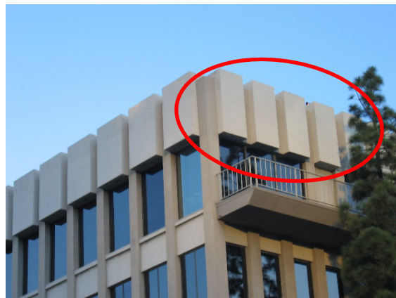
Figure 1: A well-concealed WCF. Antennas are architecturally integrated into the building.
