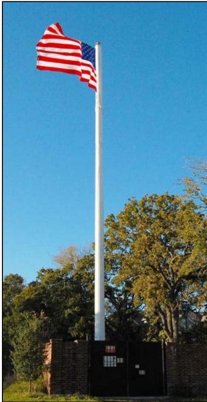
Figure 24: There are antennas in this flagpole.
