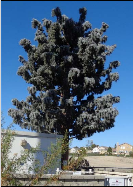
Figure 21: A mono-pine. Note how difficult it is to see the antennas.
