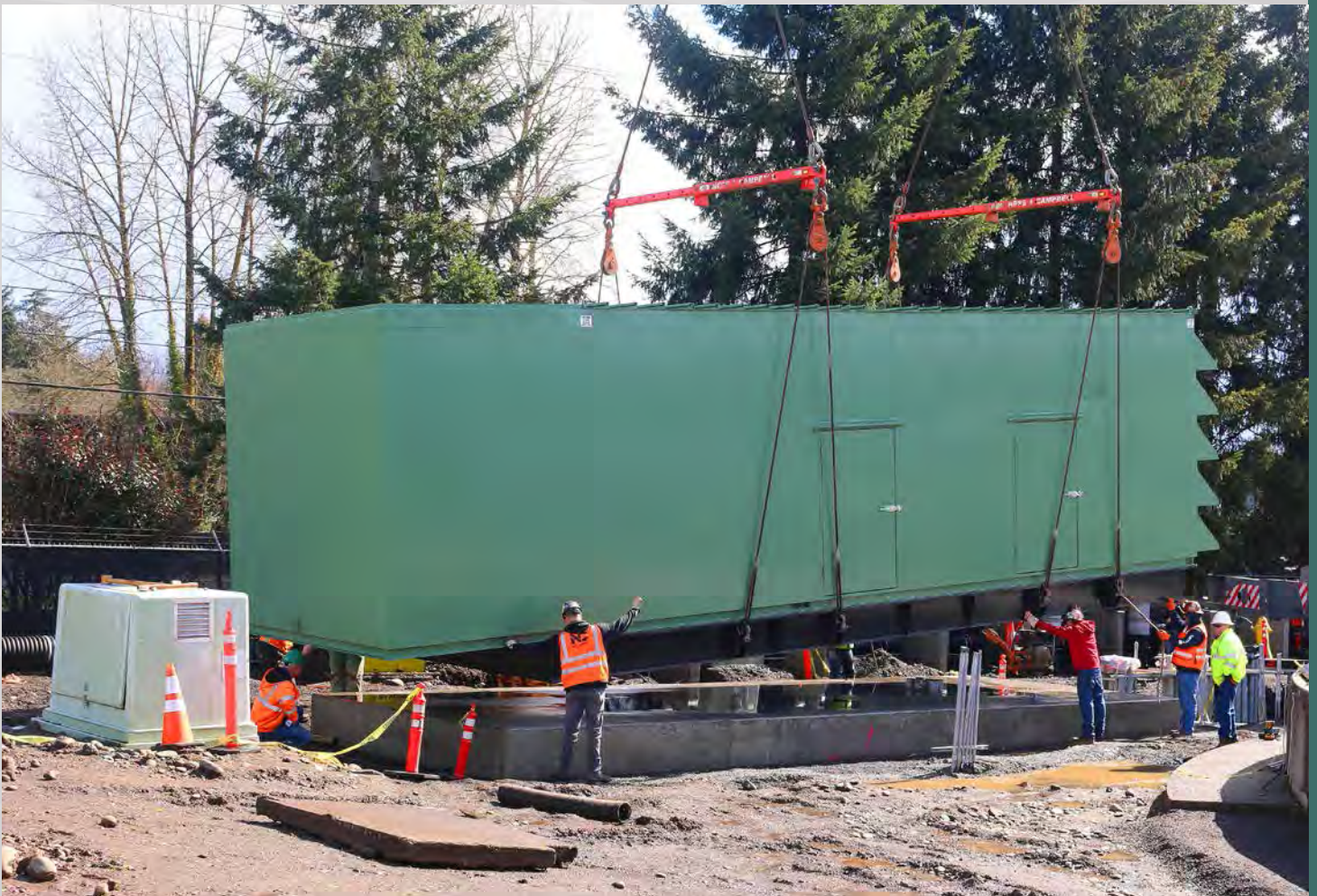
New back-up generator being placed at Kellogg Creek Water Resource Recovery Facility in Milwaukie, OR
