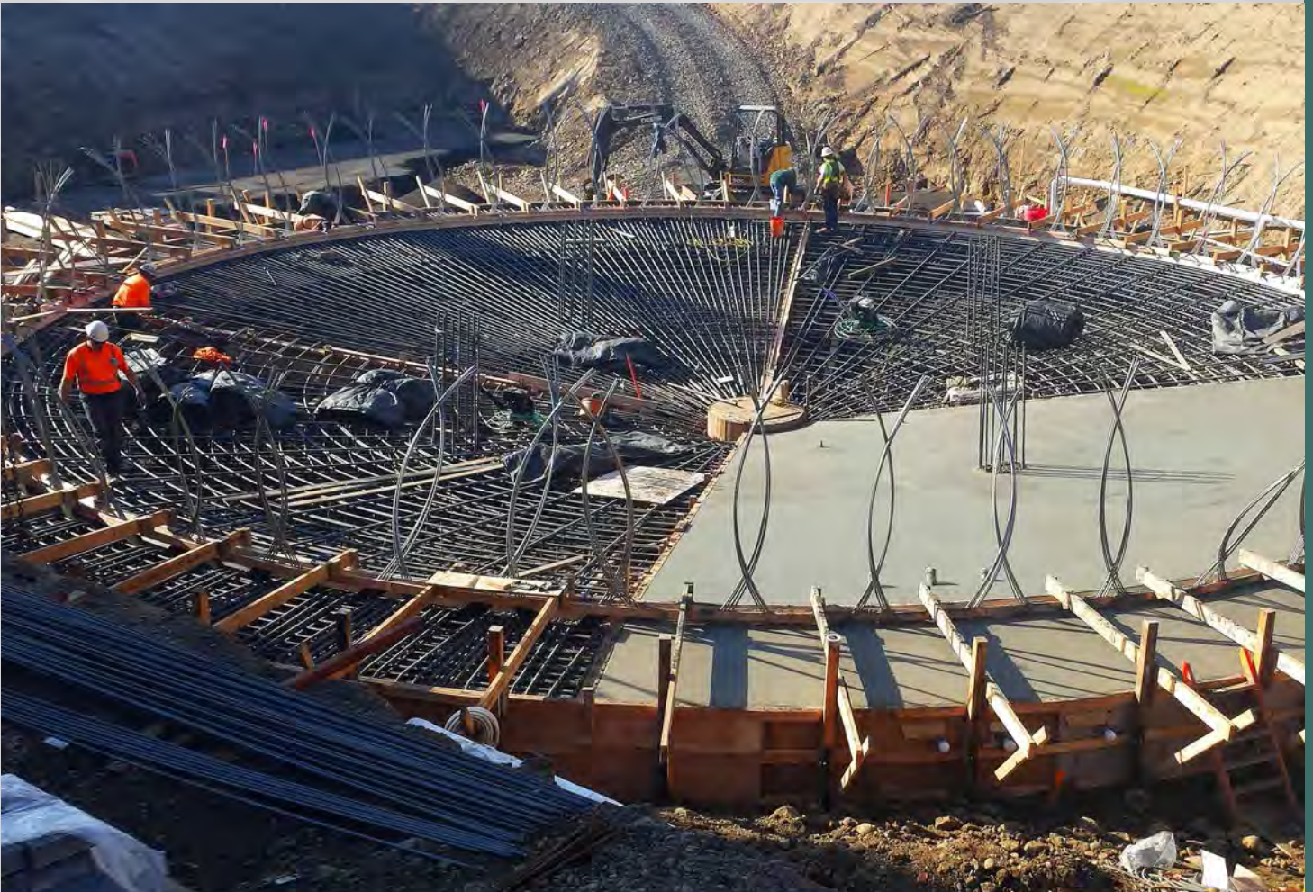
Construction of a new digester at the Tri-City Water Resource Recovery Facility in Oregon City, OR
