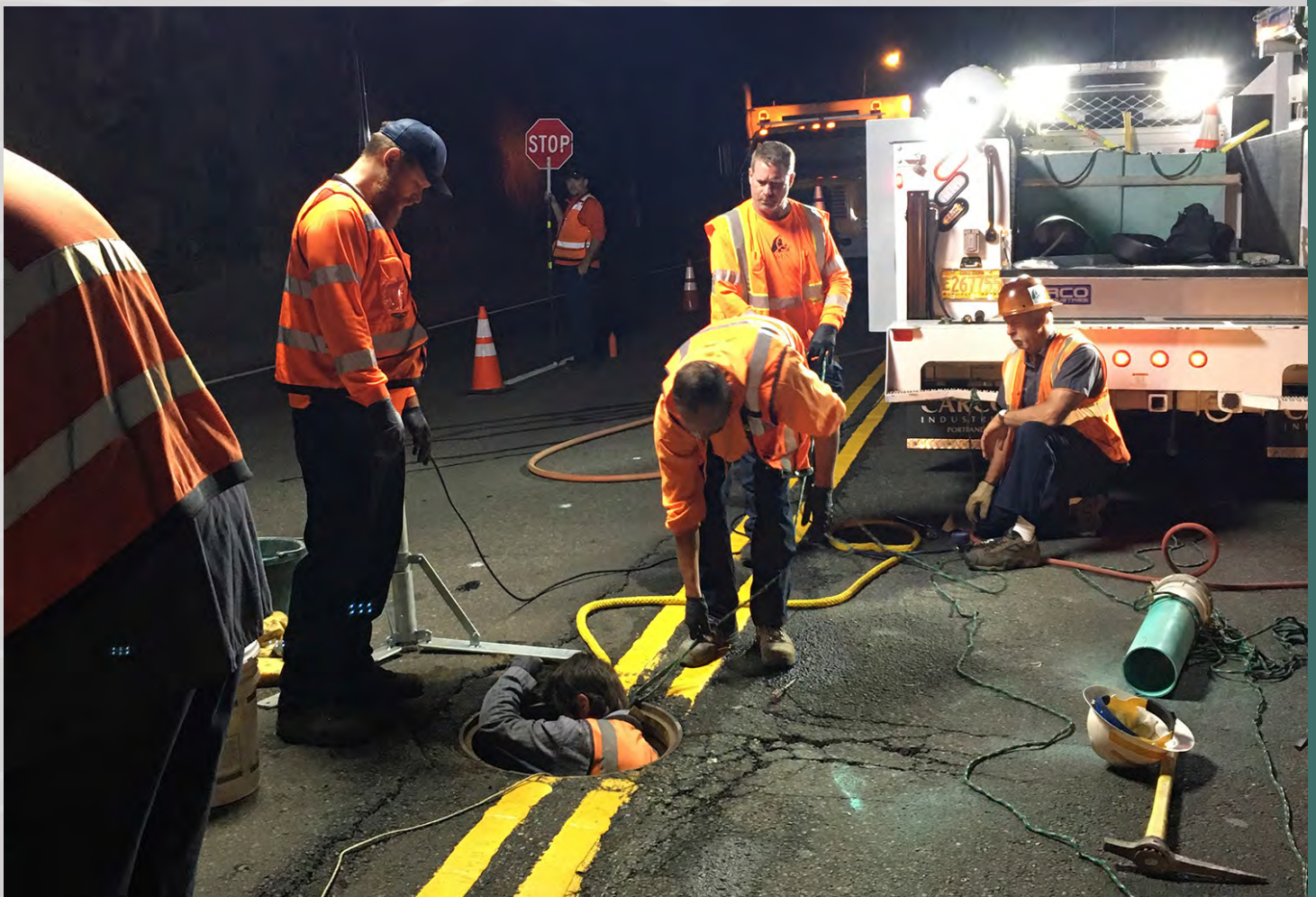
WES' field operations staff perform collection system repairs in a sewer manhole on HWY 99 in Oregon City, OR
