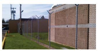
Existing perimeter fence at Jail Fence: Chain link with barbed wire, 8-foot high.
