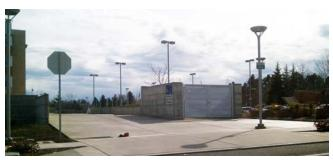
Louvered fence at DSB transformer, Courthouse Road Fence: Concrete and louvered metal panel, 12-foot high. Concrete and Mealt pane
