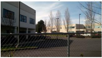
Existing chain link fencing at Silver Oak easement Fence: chain link, 4-foot high.
