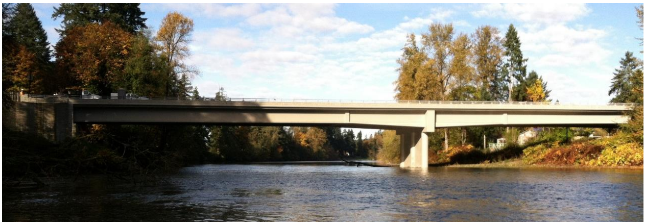
Carver Bridge (Springwater Road), after construction
