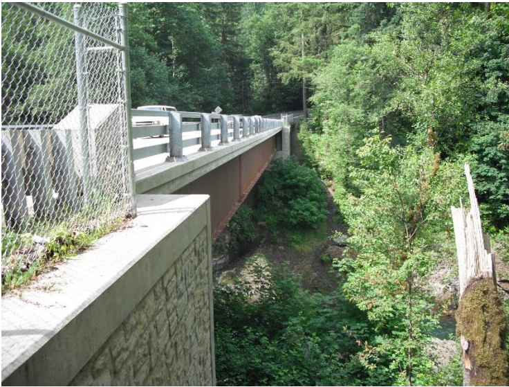
Bridge over Sandy River, after construction
