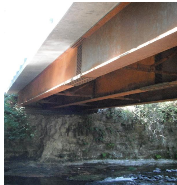
North Fork (Dickey Prairie Road), after construction
