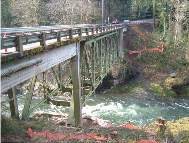
Bridge over Sandy River, before construction
