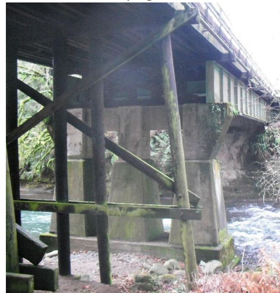
North Fork (Dickey Prairie Road), before construction
