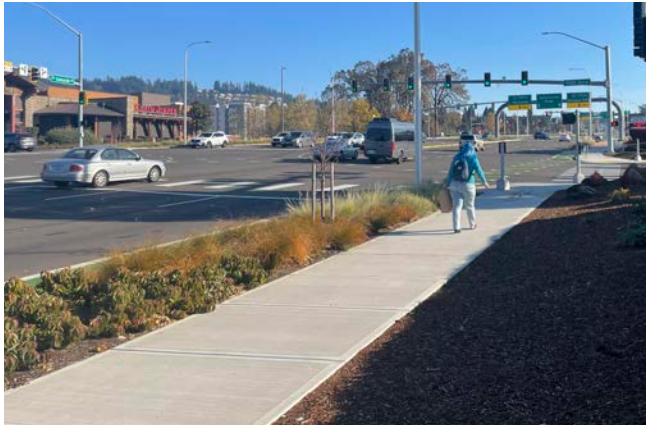
Figure 7 Sidewalks in Clackamas Regional Center Area
