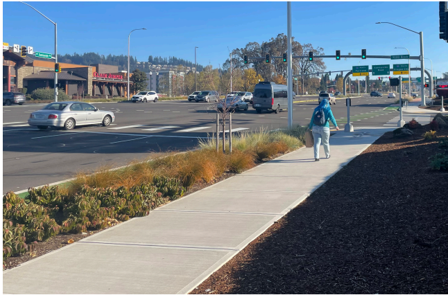
Figure 7 Sidewalks in Clackamas Regional Center Area
