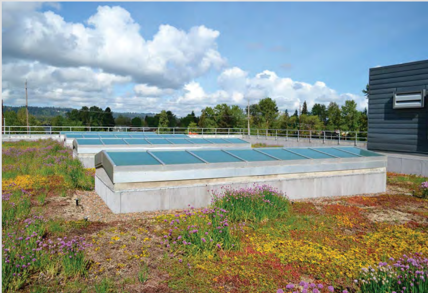
Green roof on top of the Membrane Bioreactor Building at Tri-City Water Resource Recovery Facility in Oregon City, OR
