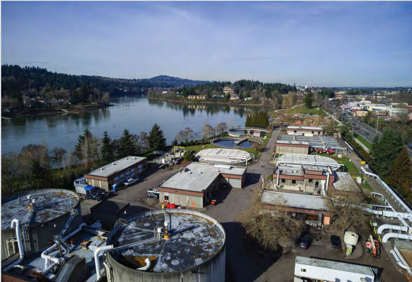
Kellogg Water Resource Recovery Facility in Milwaukie, OR
