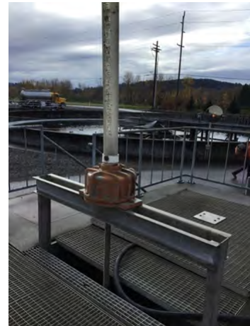
Picture 22. ML Flume No. 2 Bypass Gate
