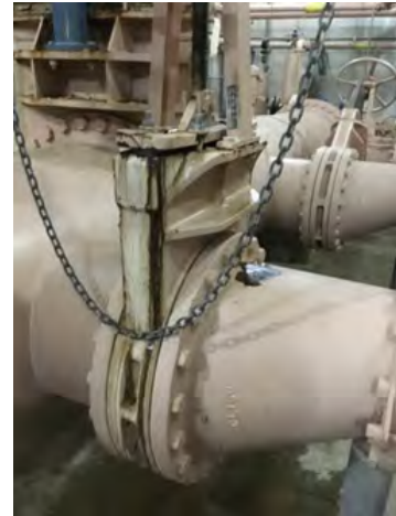
Picture 38. RAS Piping General
