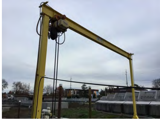
Picture 32. UV Gantry Crane
