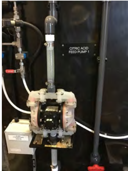
Picture 57. MBR Citric Acid Feed Pump 1
