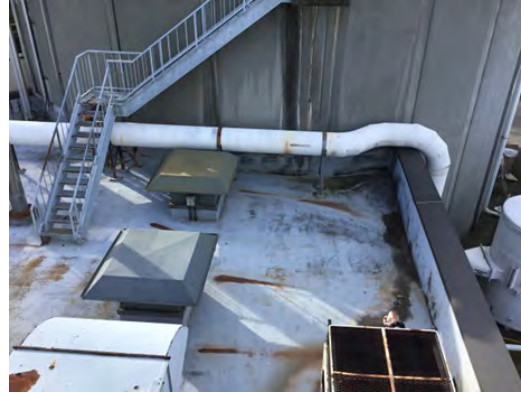
Picture 49. Digester Building (roof)
