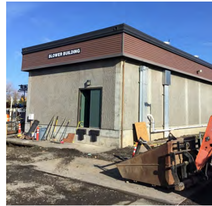
Picture 19. Blower Building
