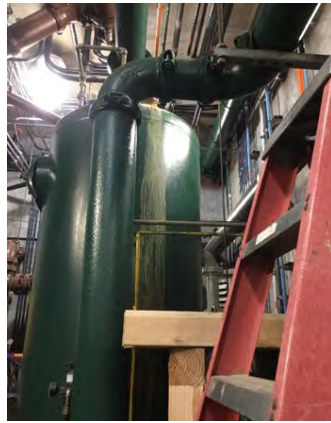
Picture 52. DAFT Air Saturation Tank
