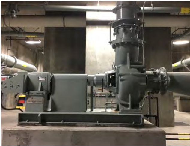
Picture 45. MBR Intermediate Pump 3
