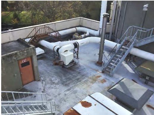
Picture 48. Digester Building (roof)
