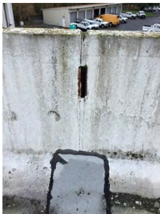
Picture 55. CAS Anaerobic Digester Tank 2
