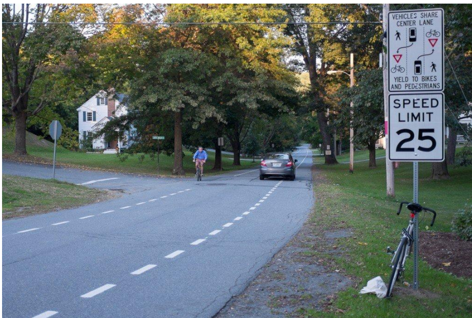
Figure 1. Advisory bike lane in Hanover, New Hampshire. Copyright 2014 The Dartmouth Company, Inc. All Rights Reserved. Reprinted with Permission.
