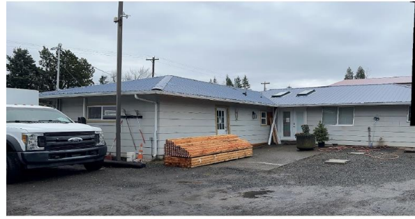
Figure 7. North-facing façade of existing structure
