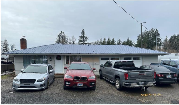
Figure 6. Front, or east-facing, façade of existing structure
