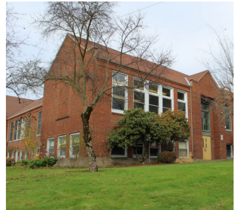
33. Exterior southeast corner
