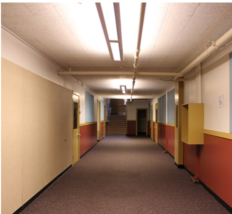
16. Lower hallway facing north
