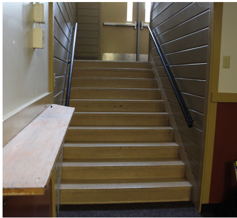
14. Northwest stair from lower level
