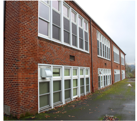
39. Exterior northwest corner
