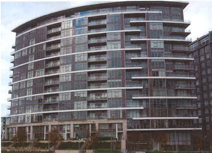
New Construction Mid-rise Condominium Portland, Oregon
