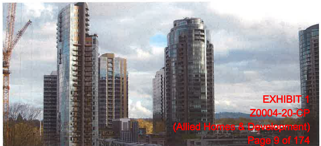
New Construction High-rise Condominiums Portland, Oregon
