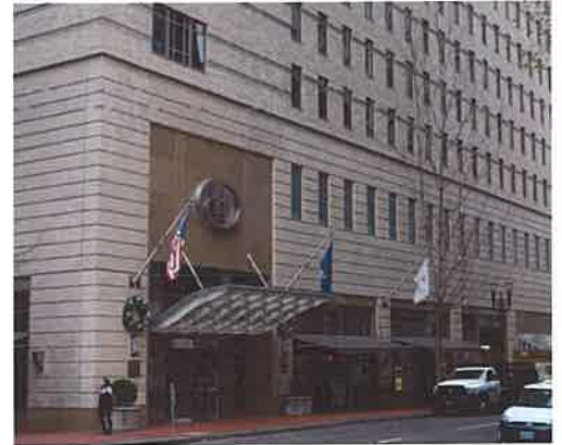
Conversion Shoebbox Condominium Portland, Oregon
