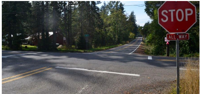
Example of roadway without shoulders (SE Tillstrom Road at SE 222 nd Avenue)
