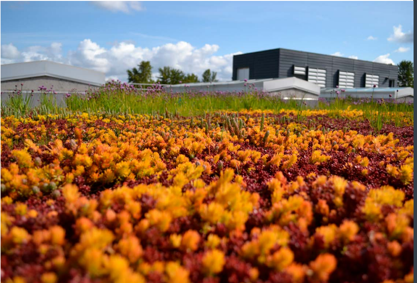
The green roof at the Tri-City Water Resource Recovery Facility
