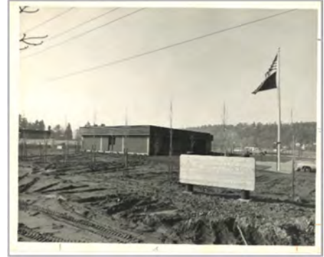
1974 - Construction of the Kellogg Creek WRRF
