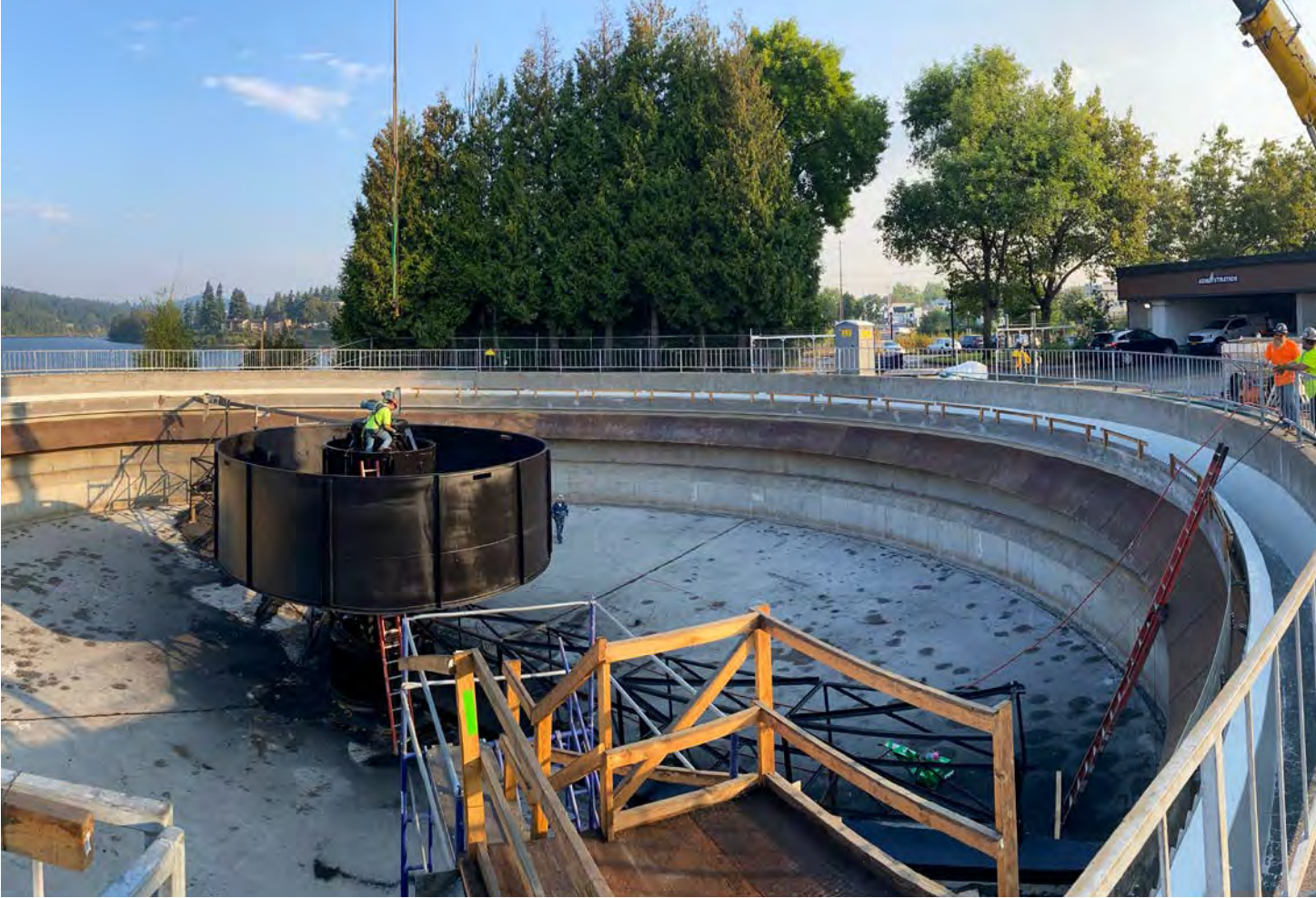
Clarifier rehabilitation at the Kellogg Creek Water Resource Recovery Facility
