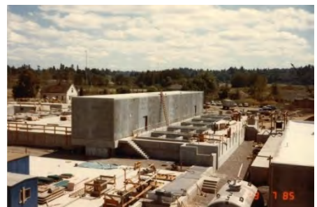
1985 – Construction of the Tri-City WRRF
