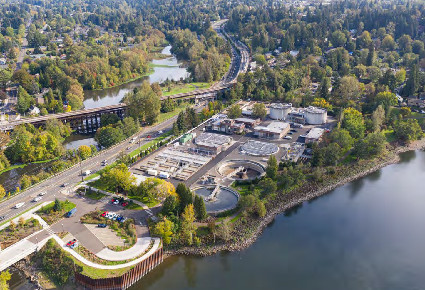
Kellogg Creek Water Resource Recovery Facility
