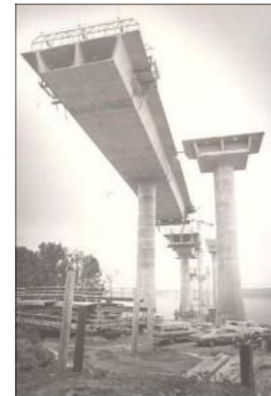
Figure 16. I-205, Glenn Jackson bridge construction in 1982
