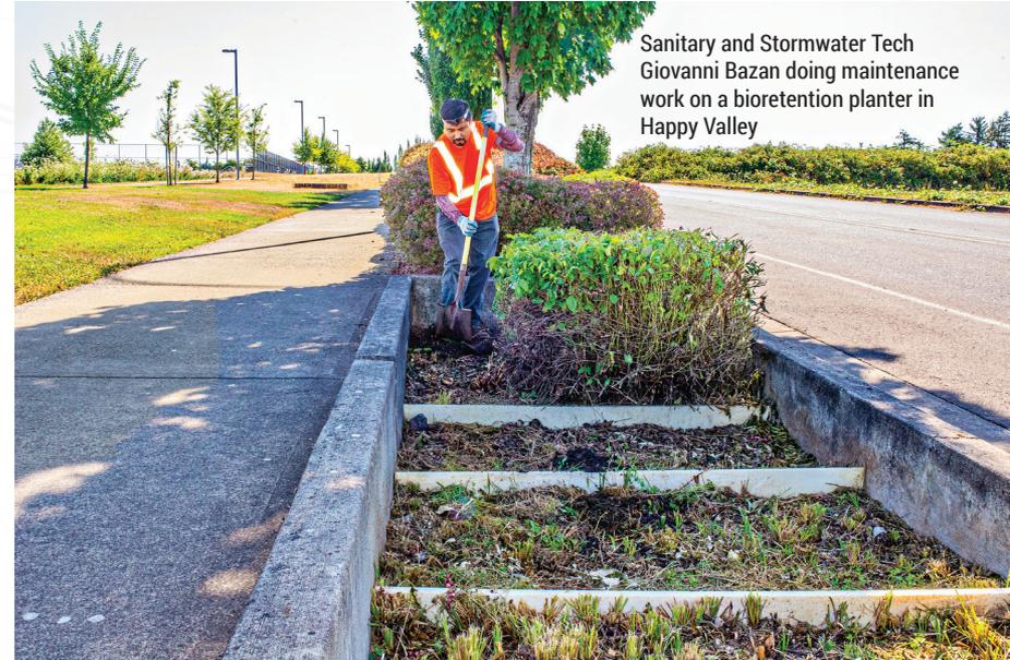
Sanitary and Stormwater Tech Giovanni Bazan doing maintenance work on a bioretention planter in Happy Valley
