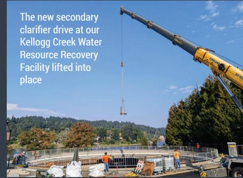
The new secondary clarifier drive at our Kellogg Creek Water Resource Recovery Facility lifted into place
