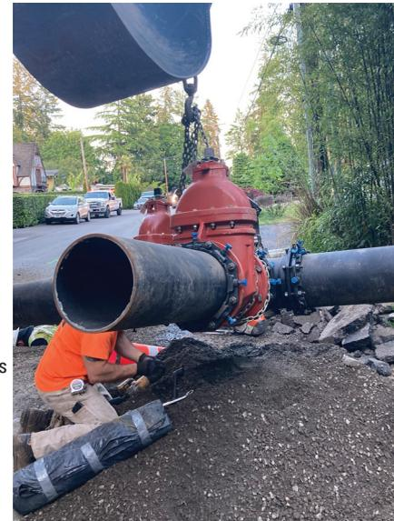
Construction crews replace an intertie valve. The work was part of the WES Pump Station Repairs and Upgrades Project, which is designed to increase reliability.
