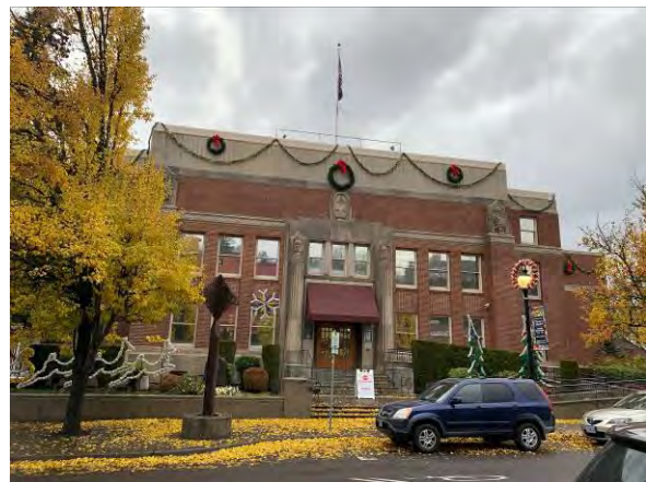
Facing northwest at subject building
