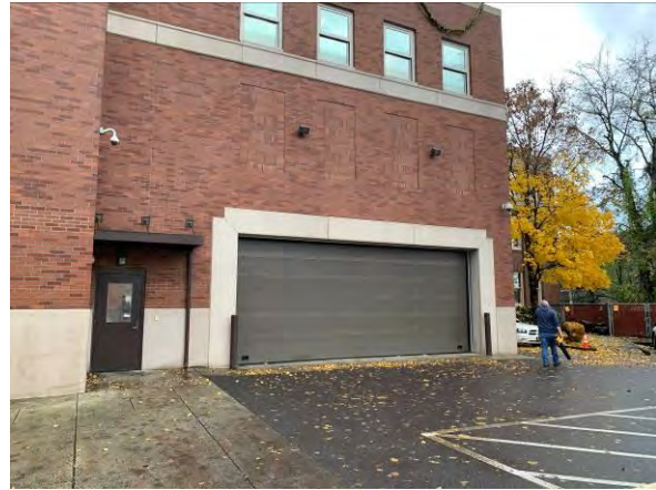
Exterior view of inmate receiving area
