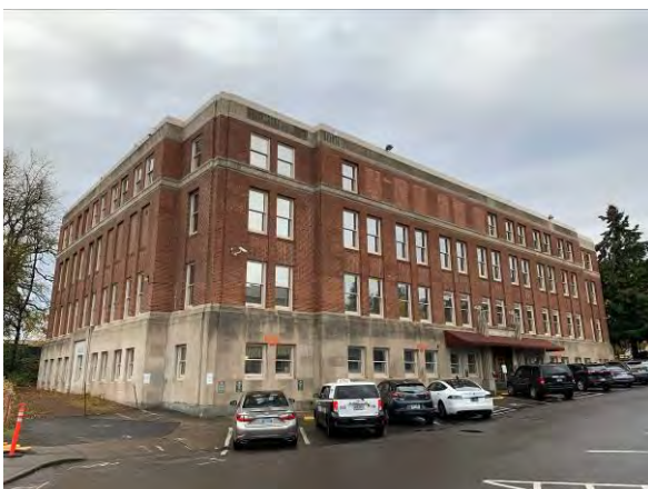
Facing east at subject building
