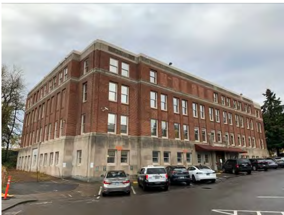
Facing east at subject building
