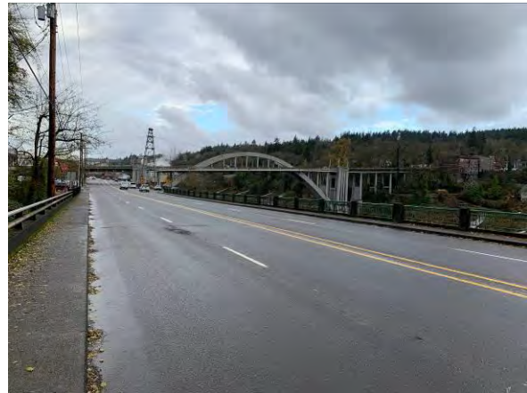
Facing southwest along Hwy 99E
