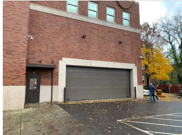
Exterior view of inmate receiving area
