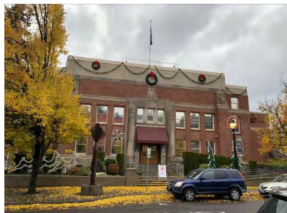
Facing northwest at subject building
