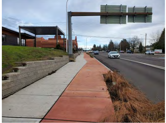
Frontage – SE Sunnyside Rd facing east
