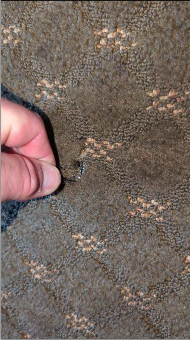
A.47. Item 5(Picture) Window seal needs repaired tear in carpet
