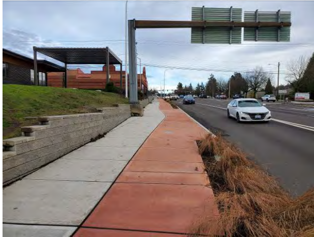
Frontage – SE Sunnyside Rd facing east
