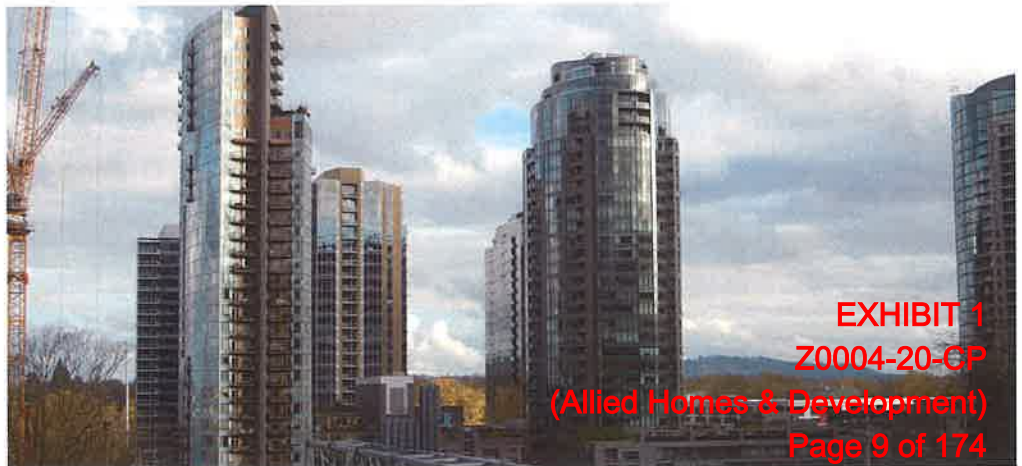
New Construction High-rise Condominiums Portland, Oregon
