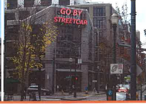
New Construction Mid-rise Condominium Portland, Oregon
