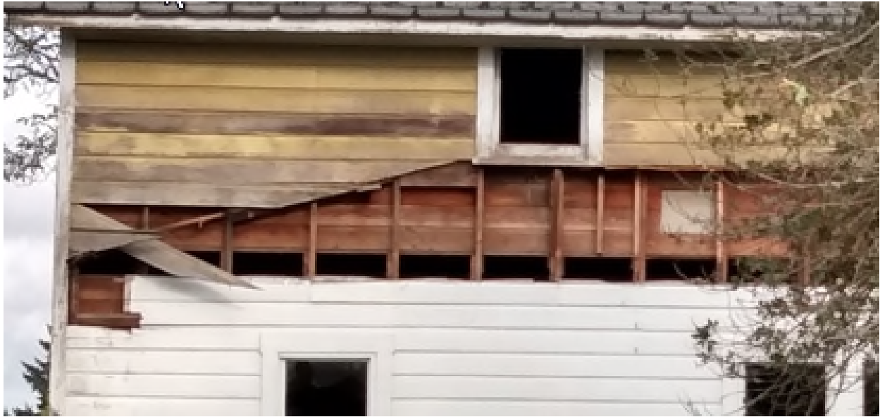
Close Up of Wall Construction
