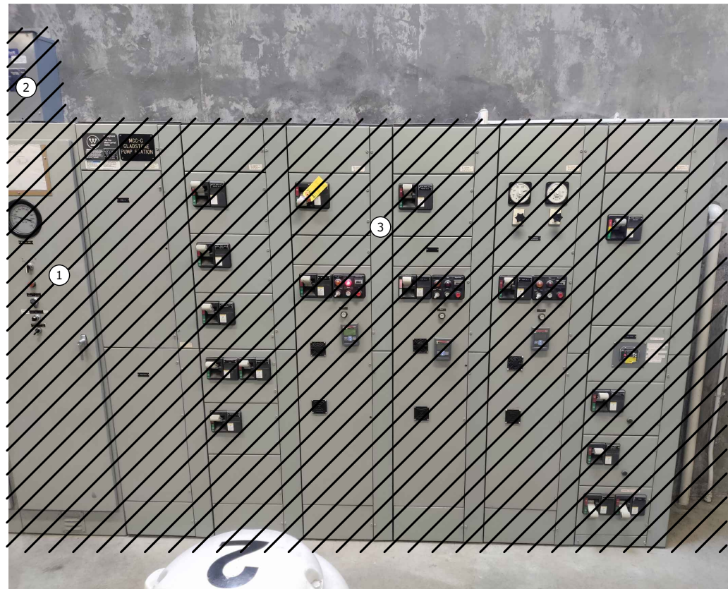
ELECTRICAL/CONTROL ROOM MCC ELEVATION
