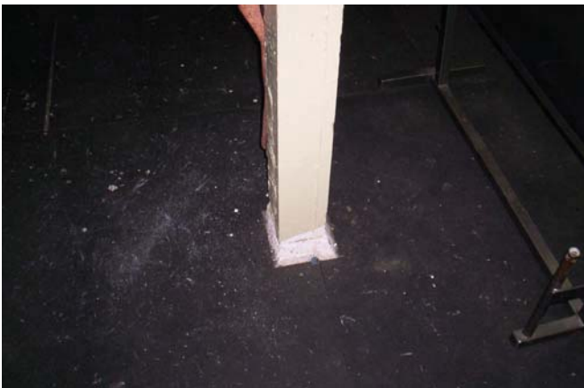
Basement post base
