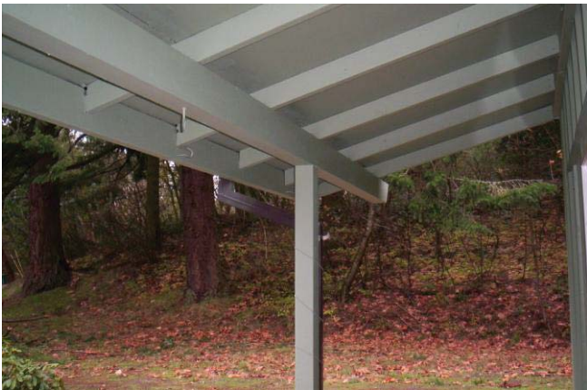
Entry Canopy Framing
