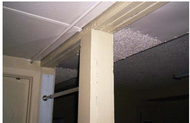
Basement post top
