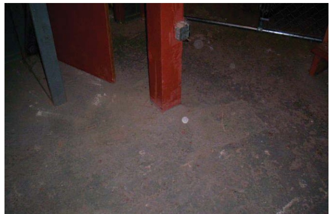
Basement post base
