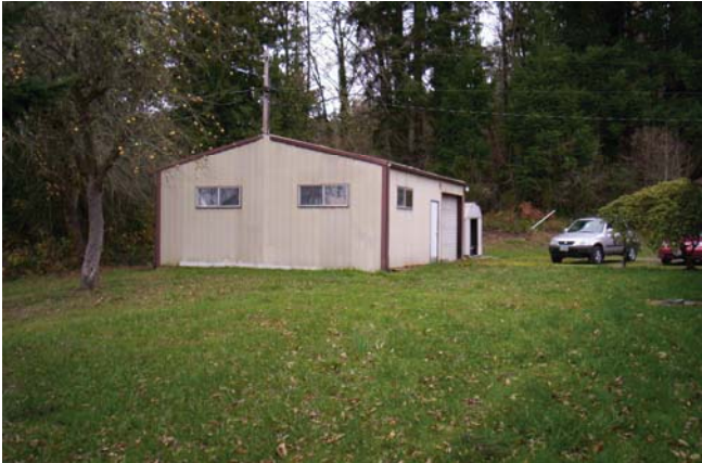
South Elevation grade at siding
