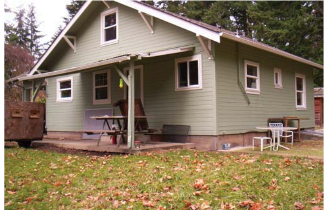
South/East Elevation with previous patio cover
