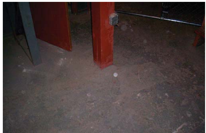
Basement post base
