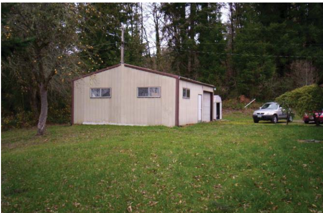
South Elevation grade at siding
