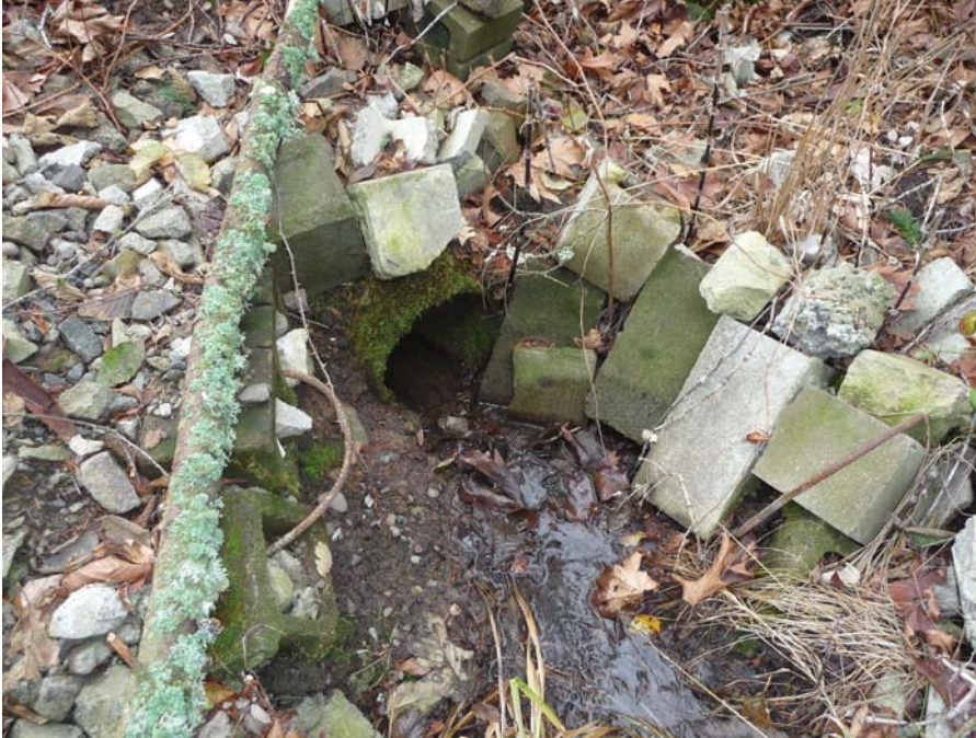
Inlet of 12" Storm line that crosses site
