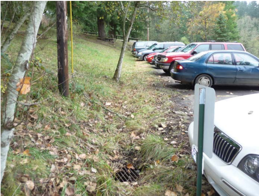
Inlet for parking area drainage
