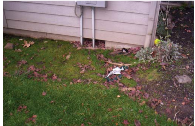
Grade at crawl space vent
