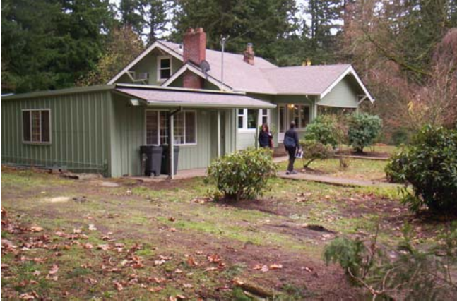
North/West Elevation with Farmhouse
