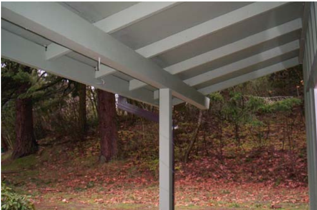
Entry Canopy Framing
